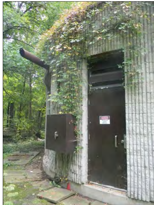
9 Looking toward the pump station entrance
