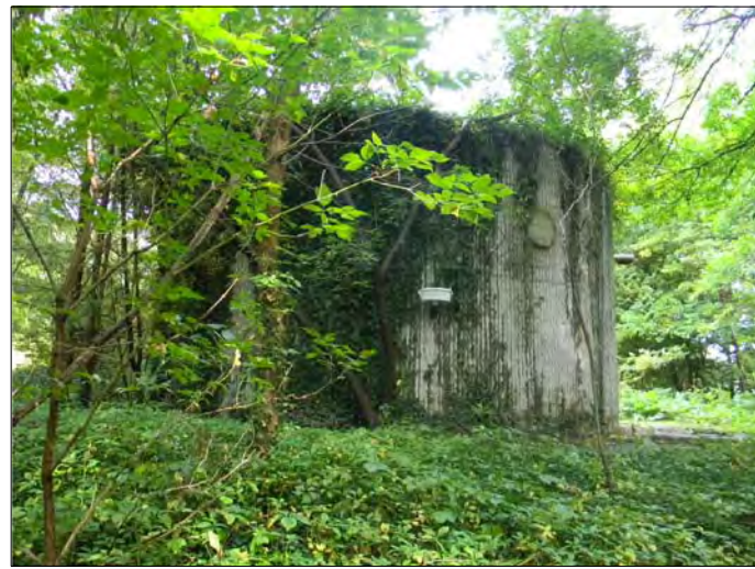
8 Looking toward the pump station from the wooded area
