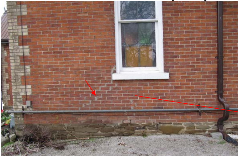
17. Some open joints in foundation. Brick generally good. Some earlier repairs at diagonal cracks.
