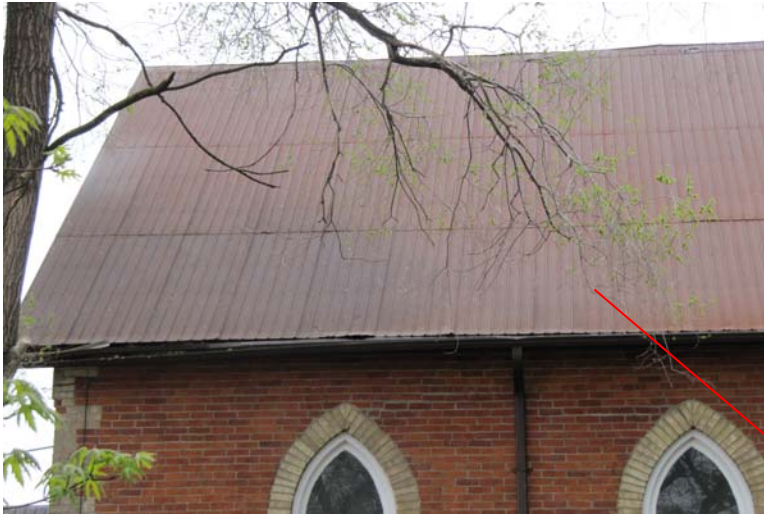
16. Roof on north side. Eavestrough falling off.
