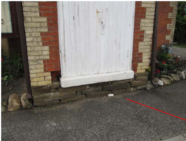
13. Unused front door. Open joints in foundation stone. Missing brick.
