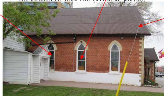
10. Window detail showing face glazed storm & condition of mid rail (peeling paint).
