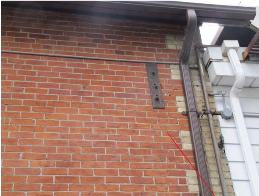
23. Steel tie rod and plate
