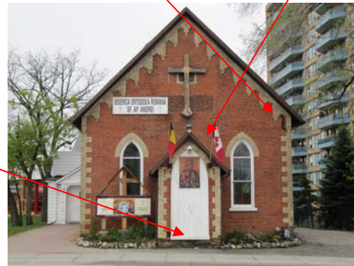
15. General view. The cross is in poor condition with open metal joints.
