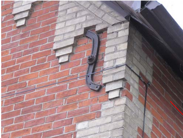
12. Steel tie. Note brick detail.
