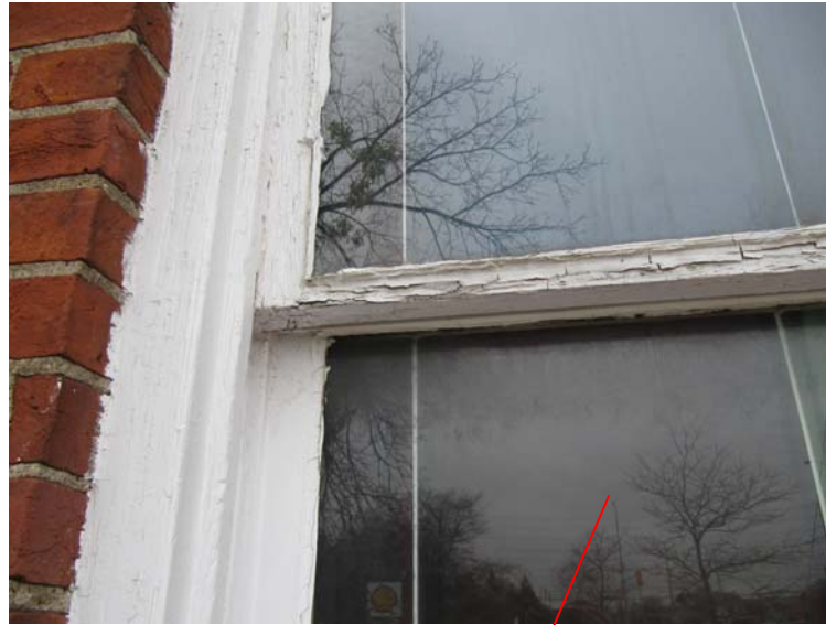
10. Window detail showing face glazed storm & condition of mid rail (peeling paint).
