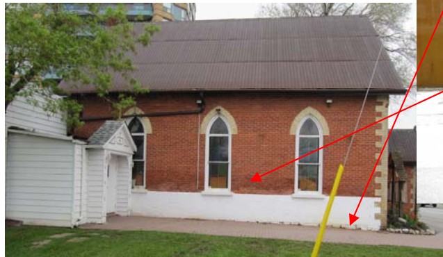
7. South side showing erosion of brick below dotted line.
