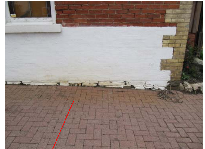
7. Painted brick. Open joints in stone foundation.
