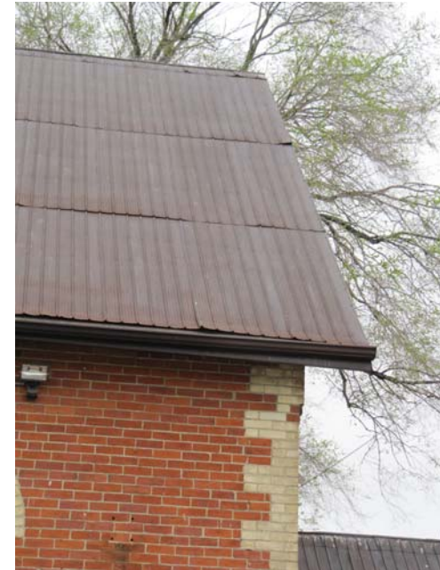
11. View showing sheets of rusty metal roof with edges curling.
