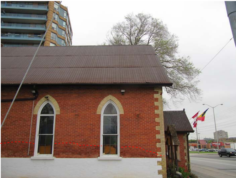
7. South side showing erosion of brick below dotted line.
