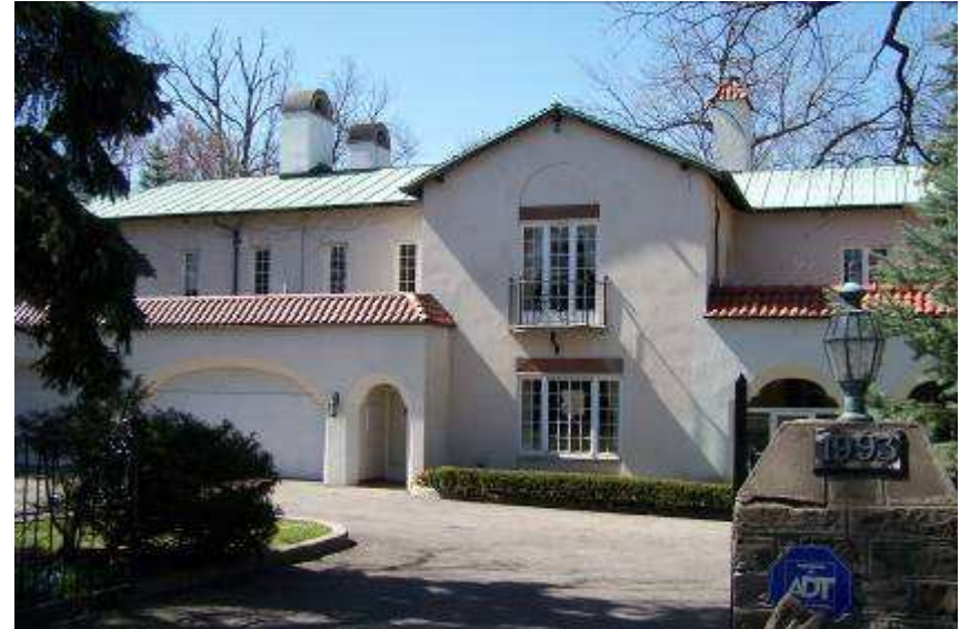
Bickell Estate , 1993 Mississauga Rd. Architects: John MacNee Jeffrey (1922) Murray Brown (1927 & 1931)
