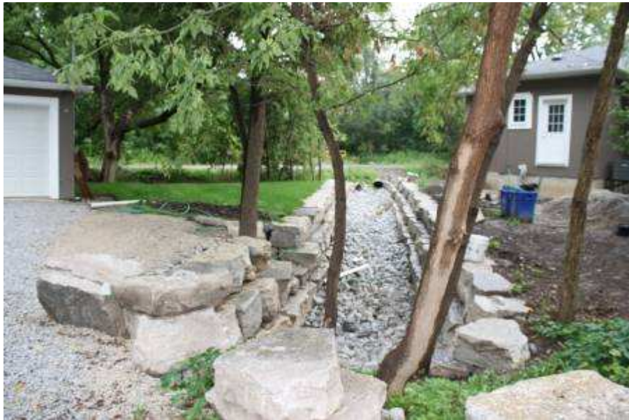
Armour stone channelled waterway from Pond Street through to Second Line West
