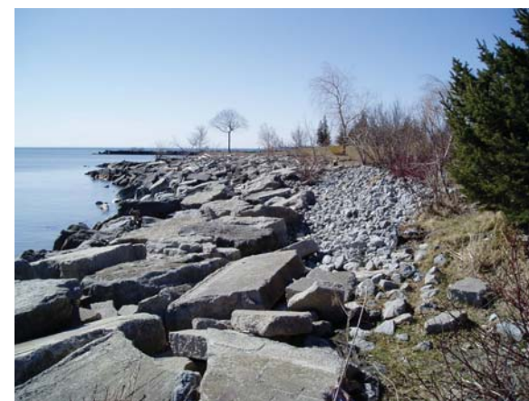
Existing dumped armourstone and riprap shoreline conditions looking west towards Imperial Oil Trail Extension.
