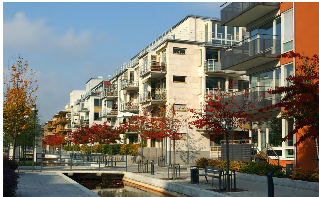
Midrise residential architecture example (Hammarby, Sweden)
