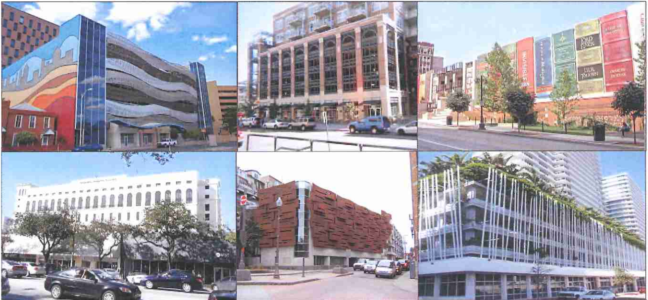
Figure 30: Facades that are articulated with architectural treatment to resemble authentic buildings, and/or more animated approaches are used to mask structured parking (applicable to 'B' Streets).
