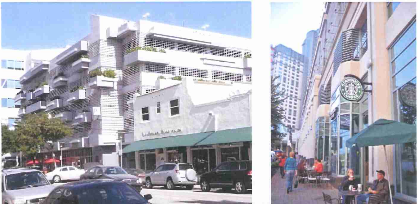
Figure 31: A typical condition for a 'B' frontage in which at grade retail is incorporated at the base and the structured parking above is enclosed by façade treatments to screen the stalls and interior parking areas.
