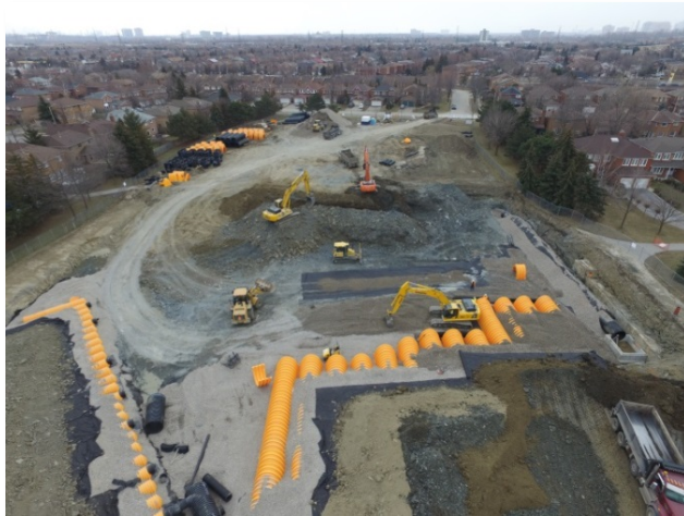
Installation of storage chambers at Eastgate Park
