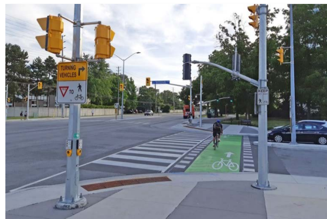
Completion of bicycle crossrides on Burnhamthorpe Road
