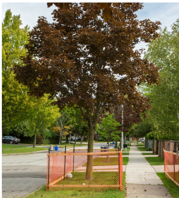
Protective Hoarding around City Tree
