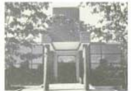
6. Dylux Distribution Centre
