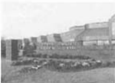
Gottardo Industrial Park
