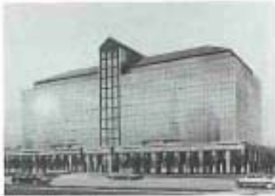
The PHH Building
