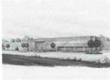
Industrial Speculative Building 245 Britannia Road East
