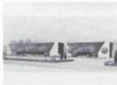
Industrial Speculative Building 6200 Tomken Road
