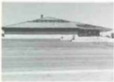
Peel Region Police Station No. 11 Division
