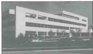
SIEMENS ELECTRIC LIMITED CANADIAN HEAD OFFICE 2185 Derry Road West
