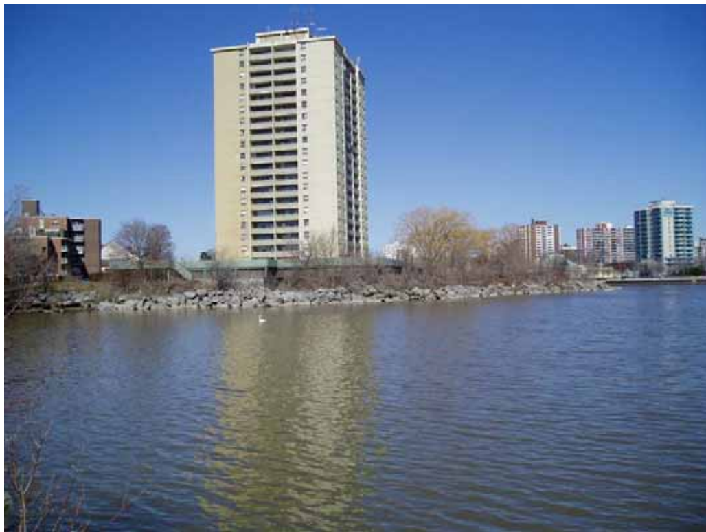
Photo A1.20 J.C. Saddington – Dumped armourstone at park extension fronting apartment
