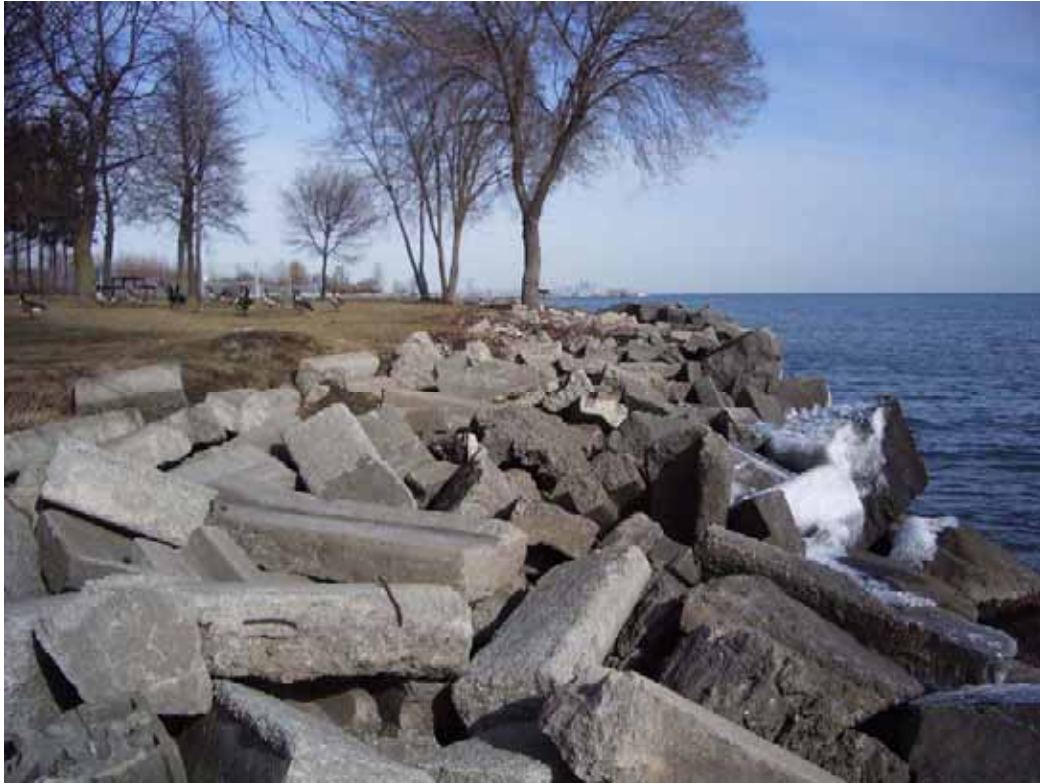
Photo A2.19 Ben Machree – Scrap concrete revetment
