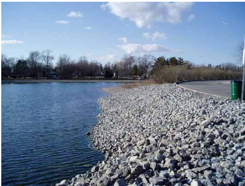
Photo A2.42 Lakefront Promenade - Riprap protection in sheltered embayment
