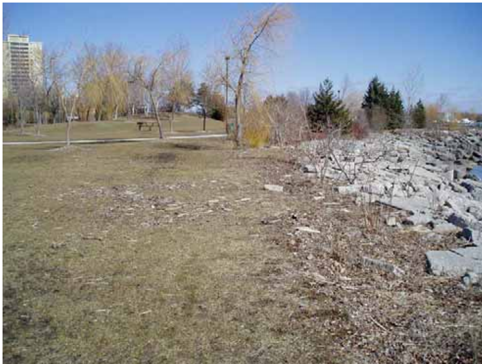
Photo A1.14 J.C. Saddington – Debris indicates runup elevation, overtopping
