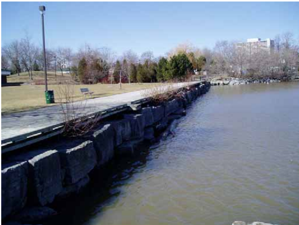
Photo A1.18 J.C. Saddington – Armourstone wall and boardwalk along credit river
