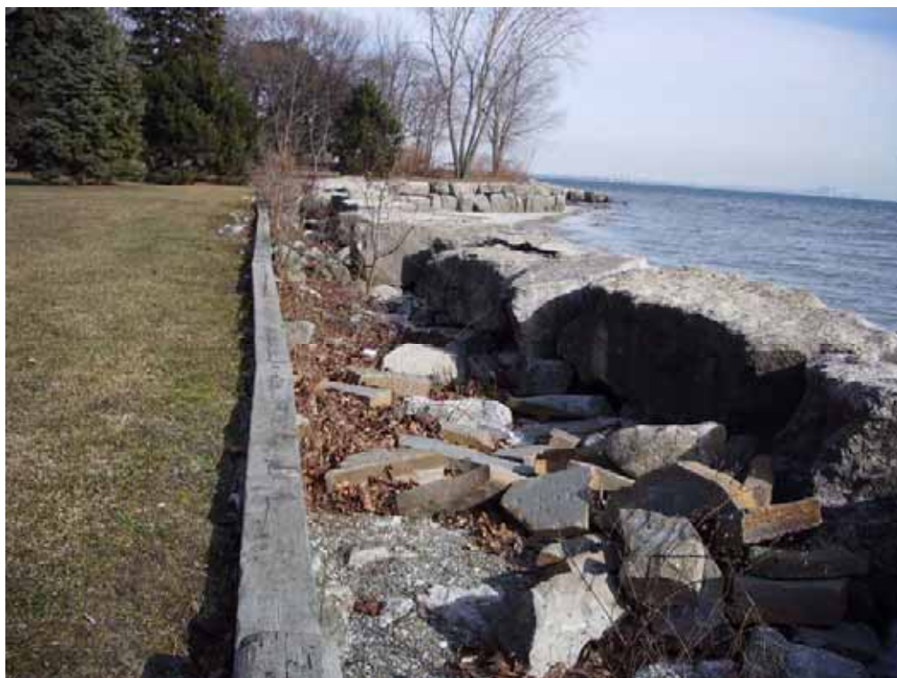
Photo A2.3 Meadowwood Park – View east showing stacked armourstone wall
