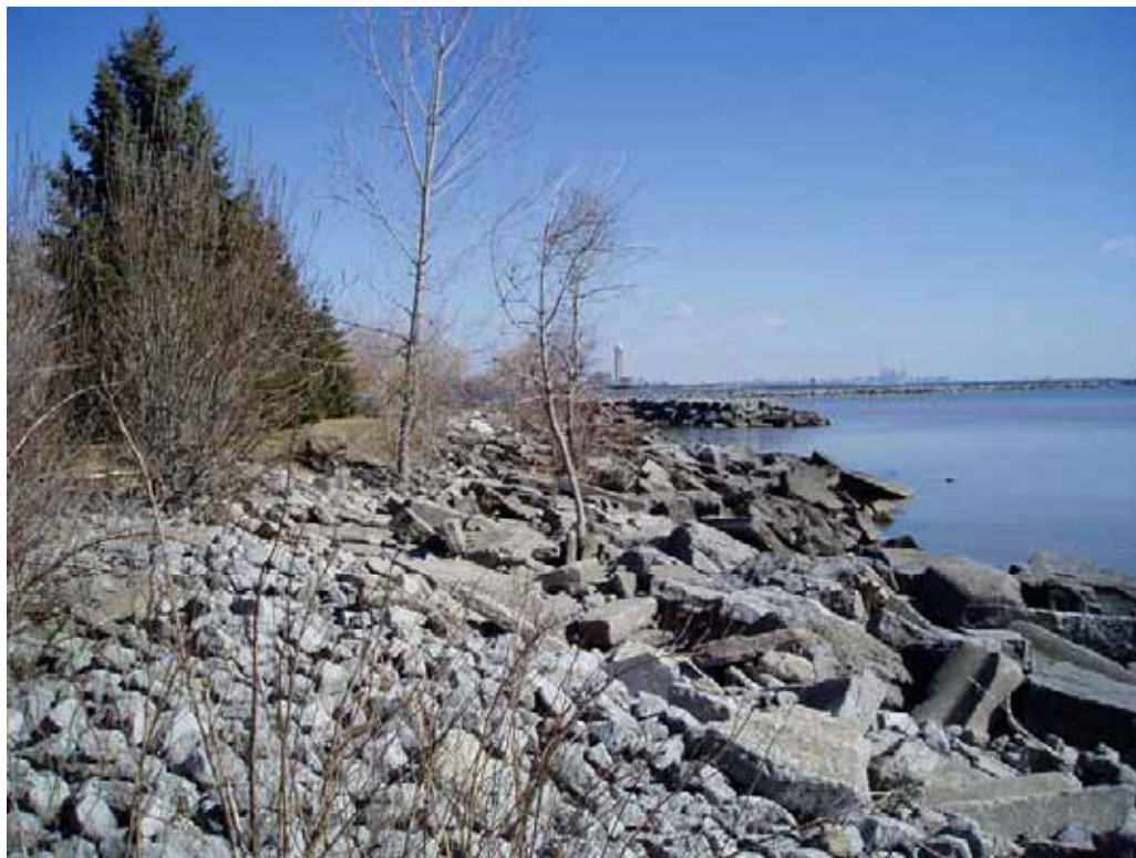
Photo A1.16 J.C. Saddington – Dumped concrete protection
