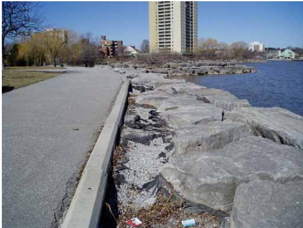
Photo A1.17 J.C. Saddington – Armourstone wall along east side of park showing exposed geotextile
