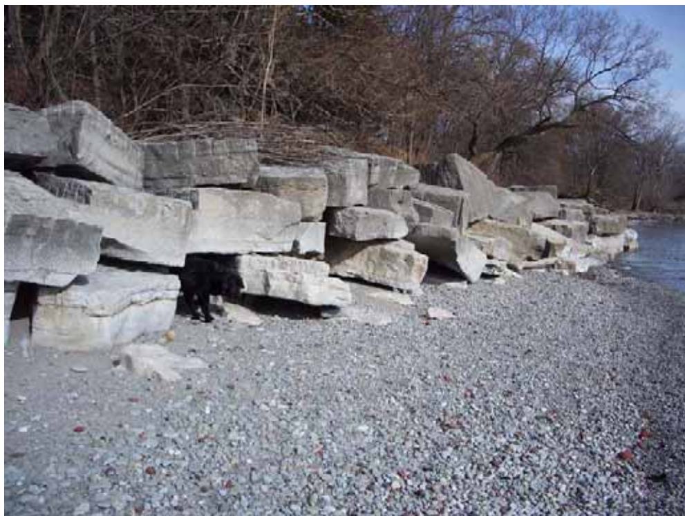
Photo A2.17 Rhododendron Park – Irregularly placed armourstone on shoreline
