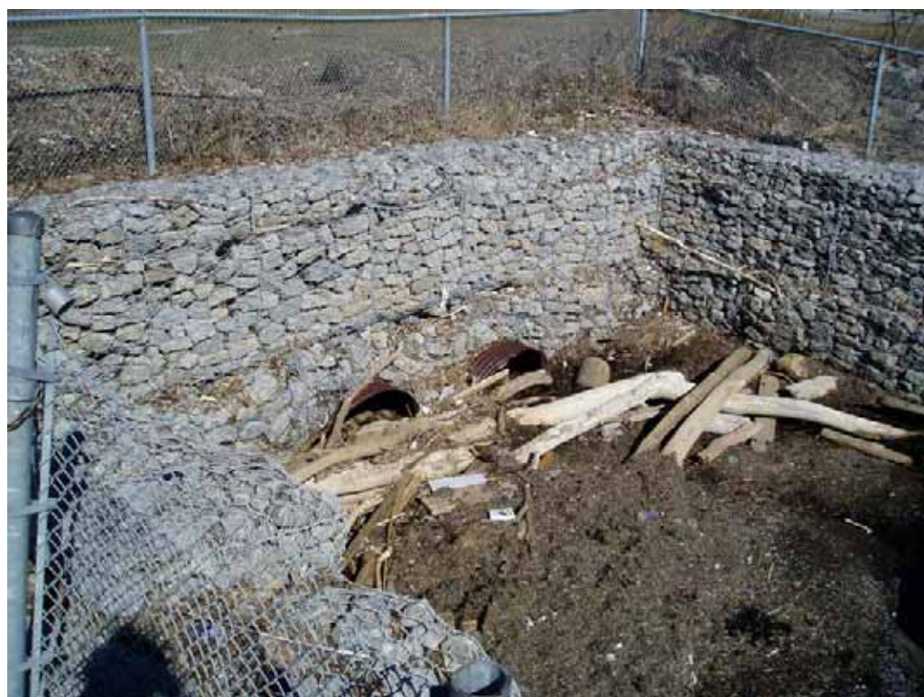
Photo A1.12 J.C. Saddington – Debris blocking culverts at west end of park
