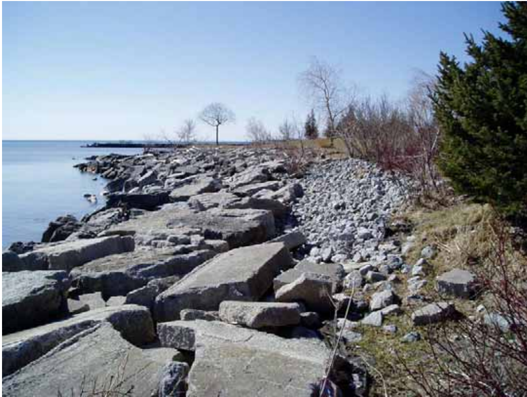
Photo A1.15 J.C. Saddington – Short term repairs include dumping riprap
