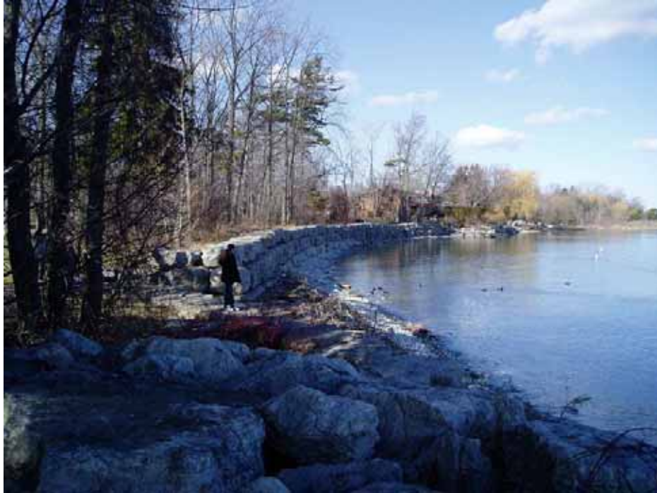
Photo A2.37 Adamson Estate – Stepped armourstone wall at east end of park
