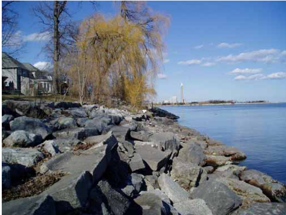
Photo A2.35 Hiawatha Park – View east along armourstone shore protection
