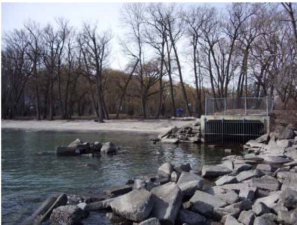
Photo A2.15 Richard's Memorial Park – Scrap concrete protecting headland in foreground, ox culvert located on west side of headland
