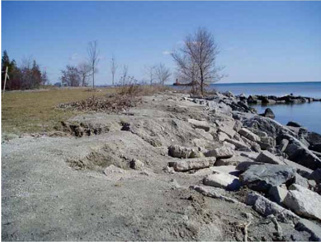
Photo A1.13 J.C. Saddington – Shoreline erosion and deteriorated shore protection
