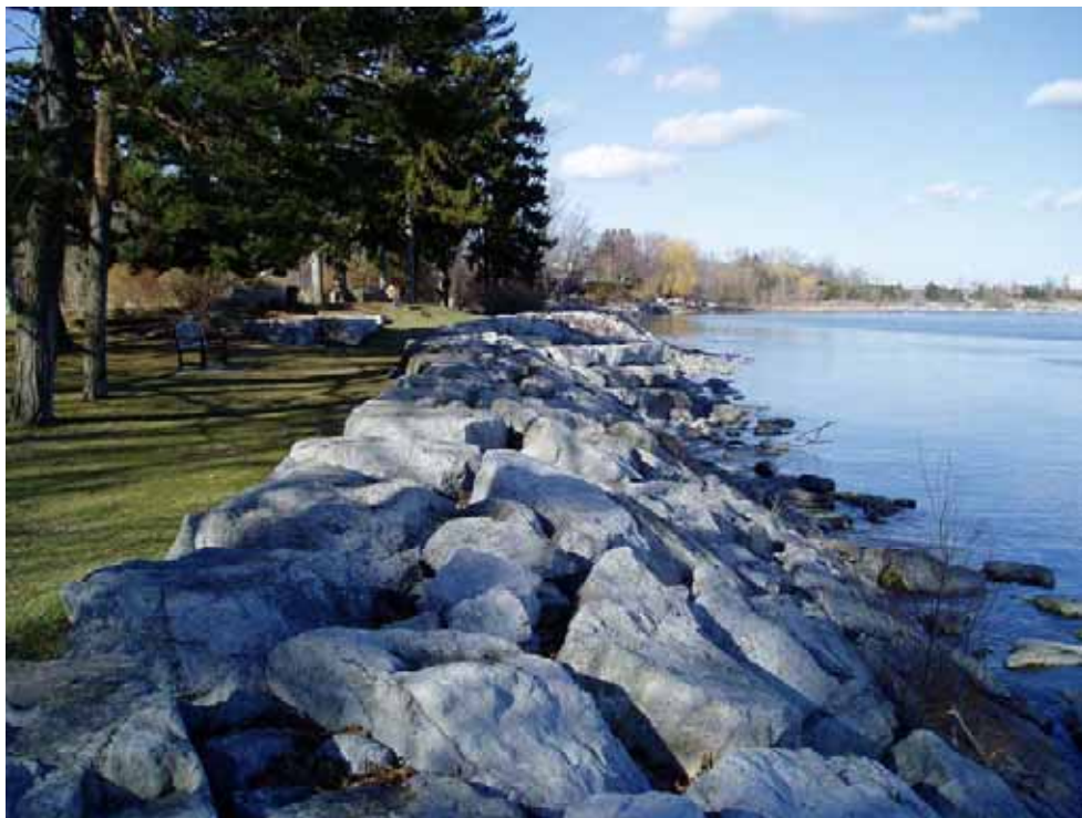
Photo A2.36 Adamson Estate – Armourstone revetment at west end of park
