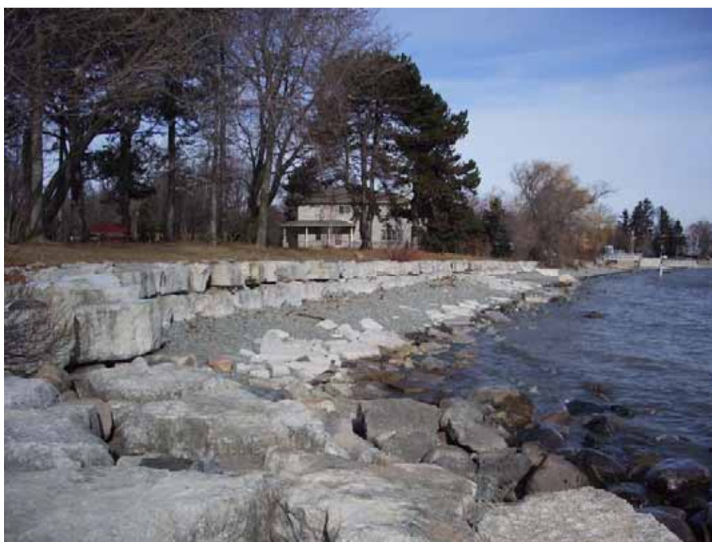
Photo A2.4 Watersedge Park – View east showing stacked armourstone wall with groyne in foreground
