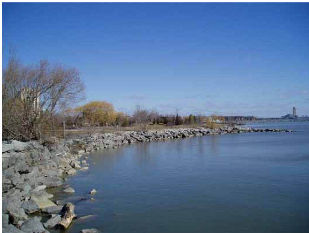
Photo A1.11 J.C. Saddington – Dumped armourstone at western limit of park
