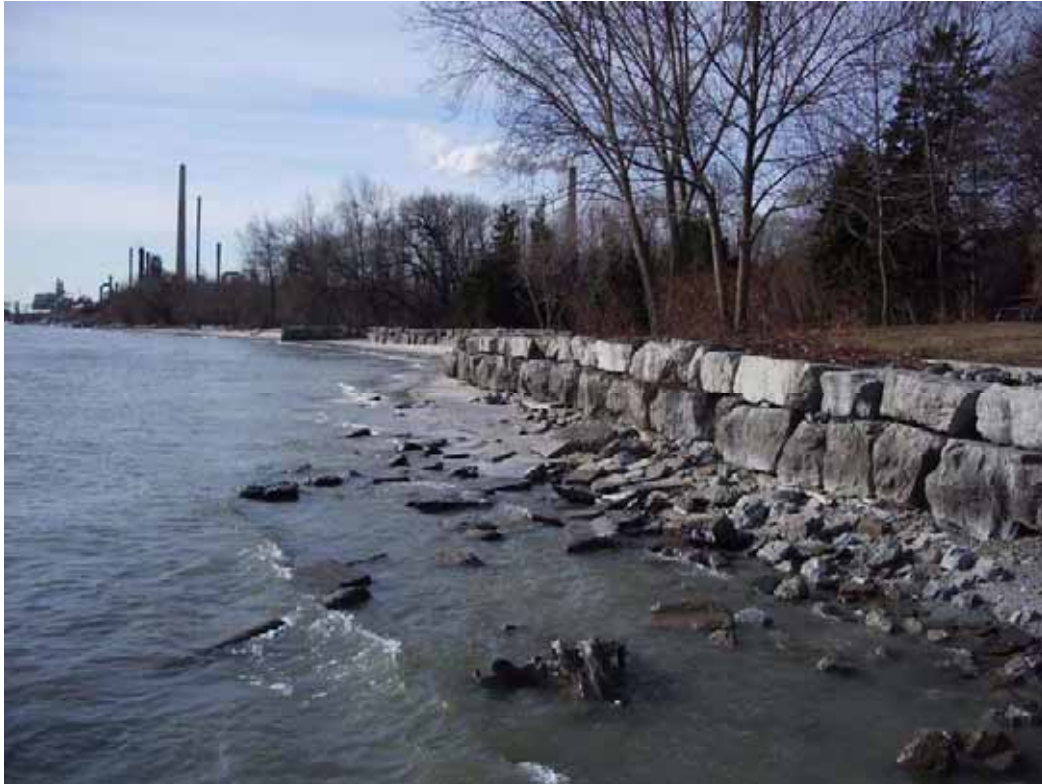
Photo A2.5 Watersedge Park – View west showing stacked armourstone wall
