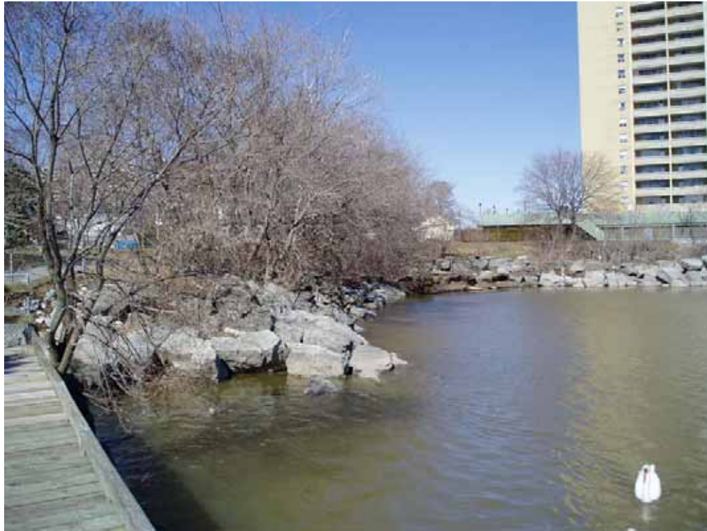
Photo A1.19 J.C. Saddington – Dumped armourstone at east end of park
