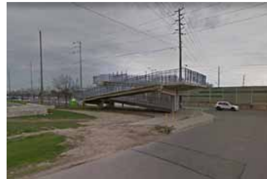
Figure V-27: Active transportation crossing of the QEW in Mississauga.
