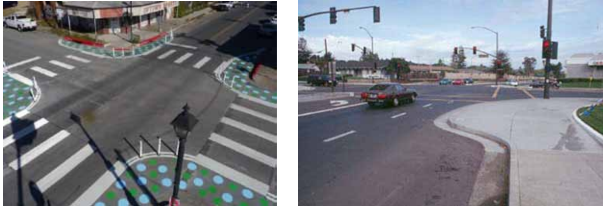
Figure V-13: Examples of curb extensions (from left to right: a) temporary treatment using paint and bollards (Austin, Texas); b) retrofitted curb extension at signalized intersection (FHWA)
