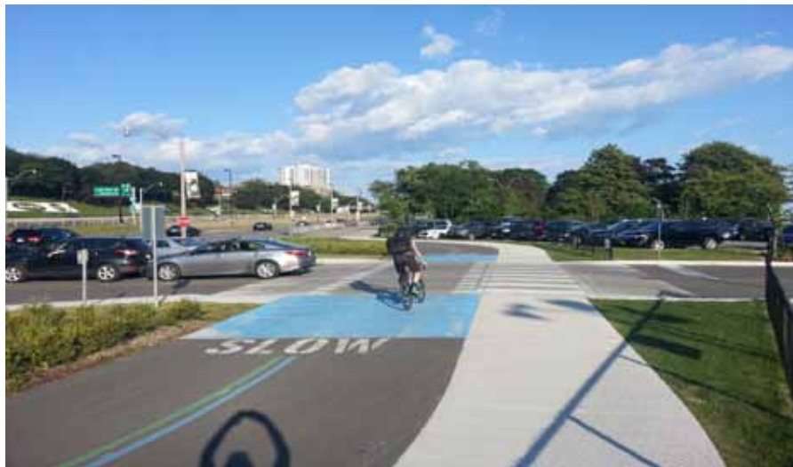
Figure V-8: Example of a recessed crossing along the waterfront trail in Toronto. The trail crossing at this busy driveway has been raised to slow motor vehicles crossing the trail.
