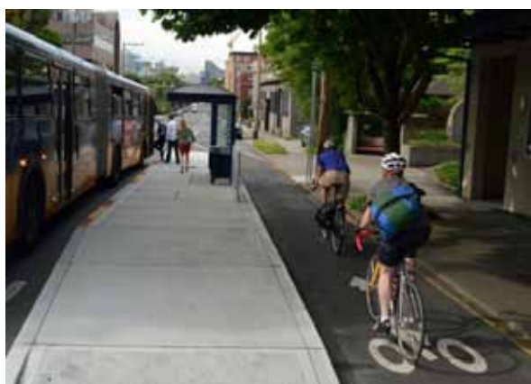
Figure V-33: “Floating” transit stops protect cyclists on a buffered bike lane in Seattle, WA (Image credit: NACTO)
