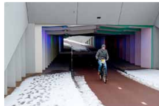
Figure V-28: Active transportation crossing of a highway in the Netherlands.
