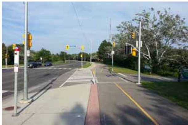
Figure V-16: Example of multi-use trail with adjacent sidewalk in Toronto. Note the use of a red tactile buffer between bicycle and pedestrian areas. As well, poles and obstacles are placed in the buffer or out of the way of the pedestrian and cycling areas.
