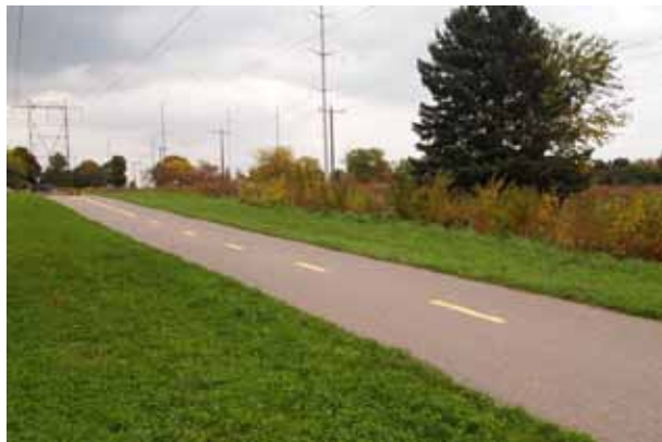
Figure V-22: Hydro corridor trail in Toronto. All new major trails in the city have centrelines.
