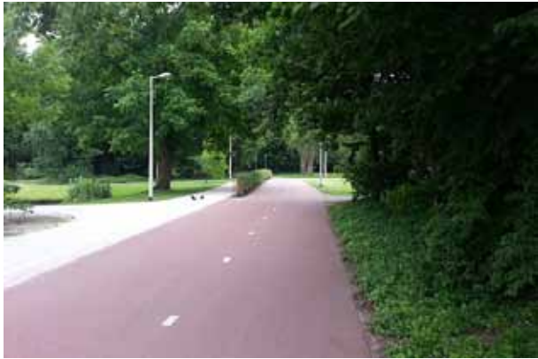
Figure V-14: Two-way bike path with adjacent pedestrian path, through a park in the Netherlands. Red asphalt and white markings are standard for all bike infrastructure in the country.
