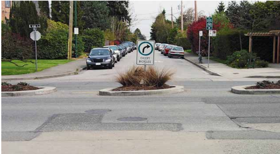
Figure V-31: A median refuge island diverter is used in Vancouver, BC to manage volume on this bicycle boulevard. (Photo credit: Richard Drdul)
