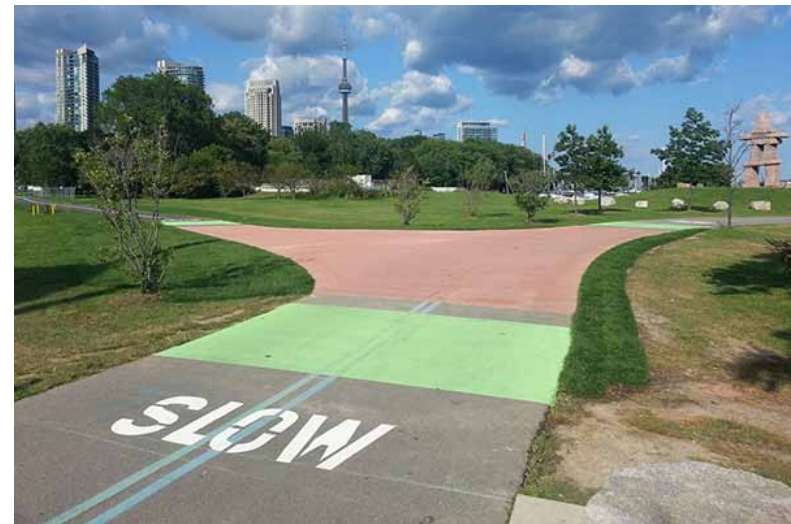
Figure V-24: Trail intersection on the Martin Goodman Trail in Toronto. The open view and wide design allows users to better navigate around each other at this location where cyclist volumes are often very high.
