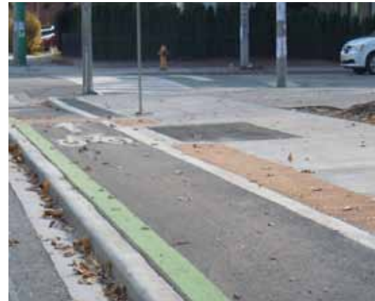
Figure V-37: Raised cycle track. In locations where the sidewalk is adjacent to the cycle track tactile pavement is used to separate the two facilities. (Image Credit: MMM, 2012)
