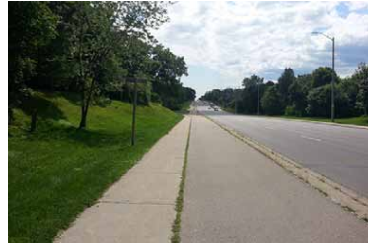
Figure V-19: A multi-use trail in Mississauga, on Lakeshore Road West. This is an example of an easy conversion to a two-way cycle track, due to an existing adjacent sidewalk. Pavement markings and intersection improvements would be needed for the conversion.
