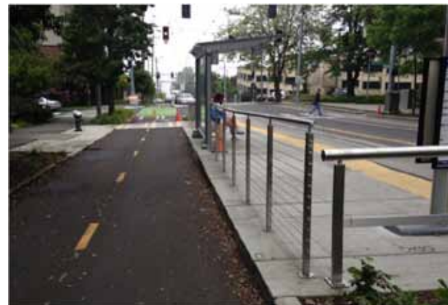
Figure V-39: A two-way cycle track with floating transit stop. (Image Credit: Dongho Chang)
