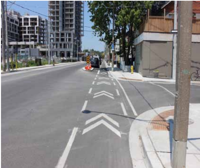
Figure V-1: This parking protected bike lane has restricted parking near to the intersection and includes pavement markings through intersections to indicated the correct positioning and priority for cyclists. (Image credit: Fred Sandoval)
