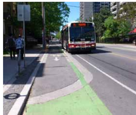
Figure V-38: A shared cycle track transit stop may be an appropriate retrofit on constrained transit routes. (Image Credit: Payton Chung)
