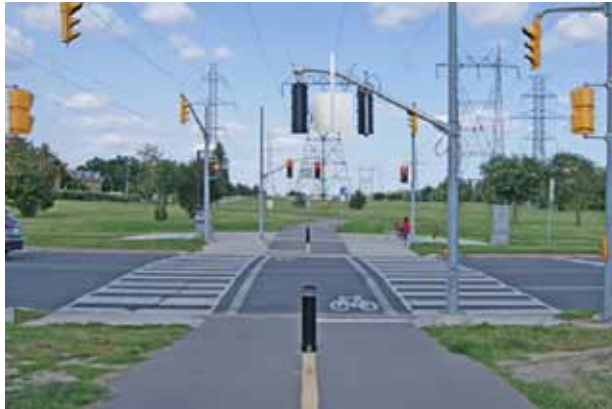
Figure V-25: Single bollard used for vehicle access control on the Finch Hydro Corridor Trail.
