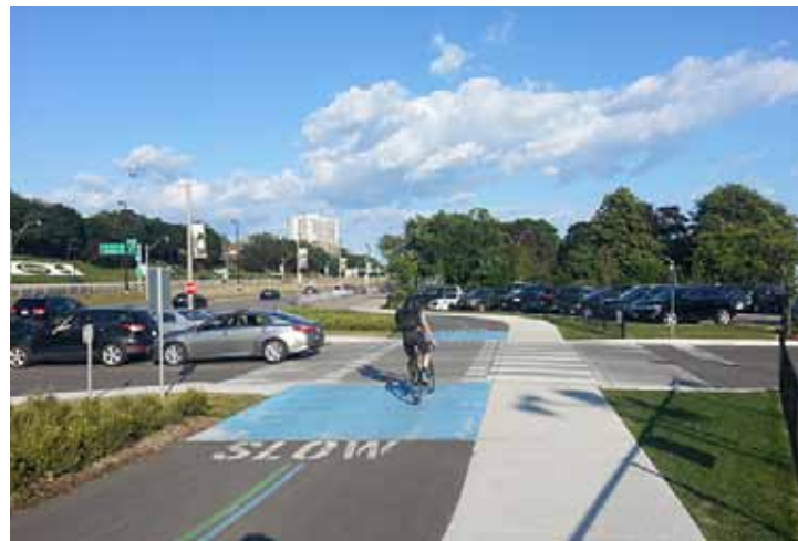
Figure V-23: Separated multi-use trail with adjacent pedestrian area, in Toronto. The blue and green lines provide branding and wayfinding for the Martin Goodman Trail/ Waterfront Trail.
