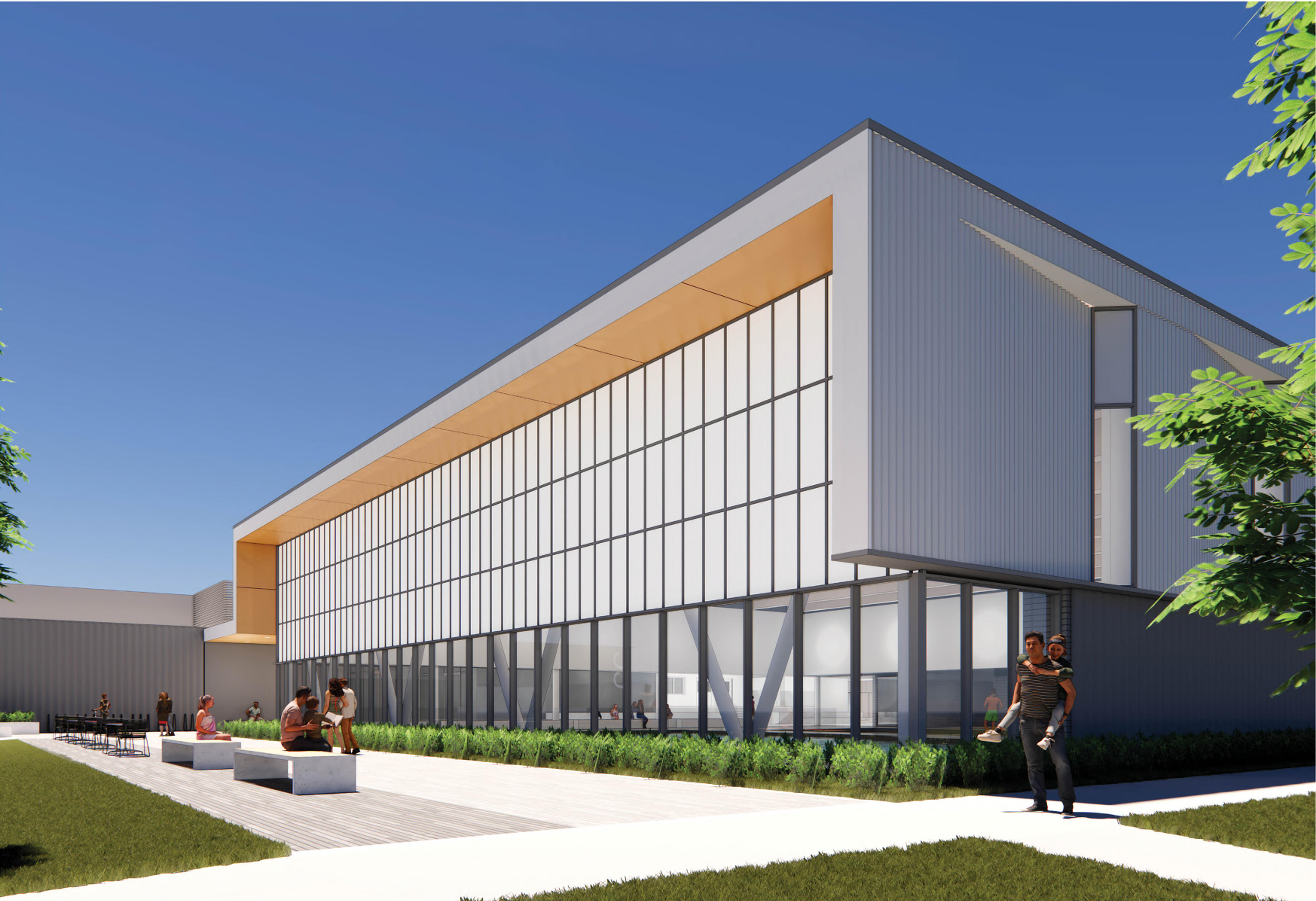
View of North-East Corner
