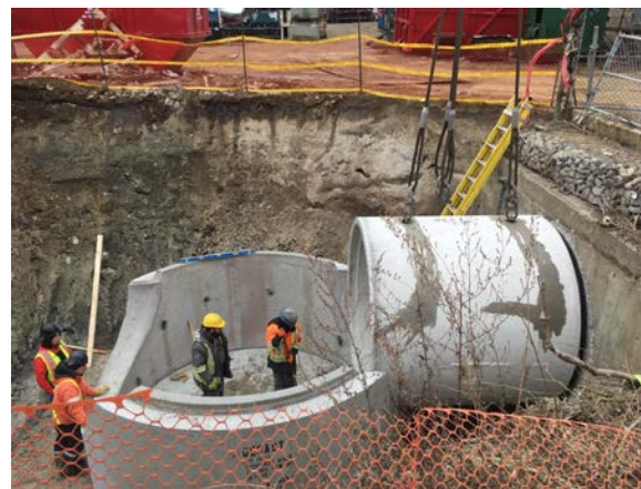
Installation of new storm pipe infrastructure (Timberlea Boulevard at Little Etobicoke Creek)
