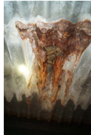
Corroded metal storm sewers require replacement
