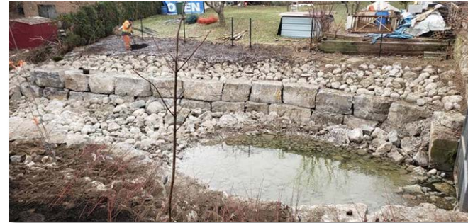
Bank protection at storm sewer outfall to Applewood Creek
