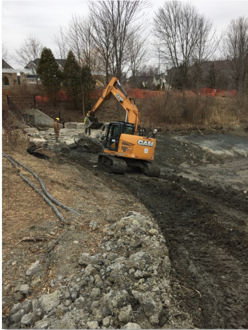
Sediment Removal from Stormwater Management Ponds
