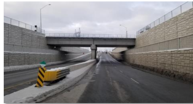
Completion of Torbram Road grade separation
