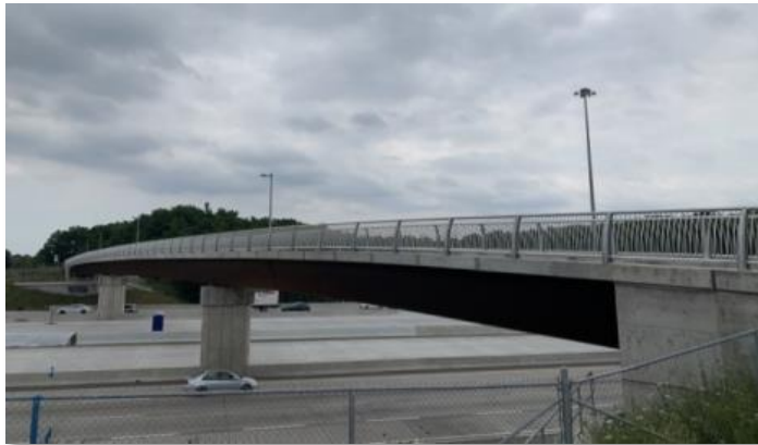
Second Line West Active Transportation Bridge over Highway 401
