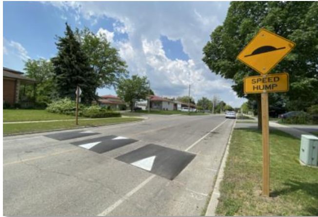
Traffic calming on Redstone Road
