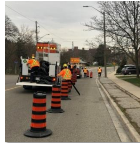
Installation of temporary Active Transportation Lane on King Street in Cooksville
