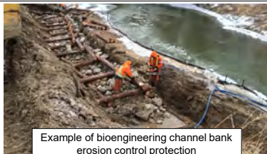
DETAIL: VEGETATED ROCK REVETMENT
