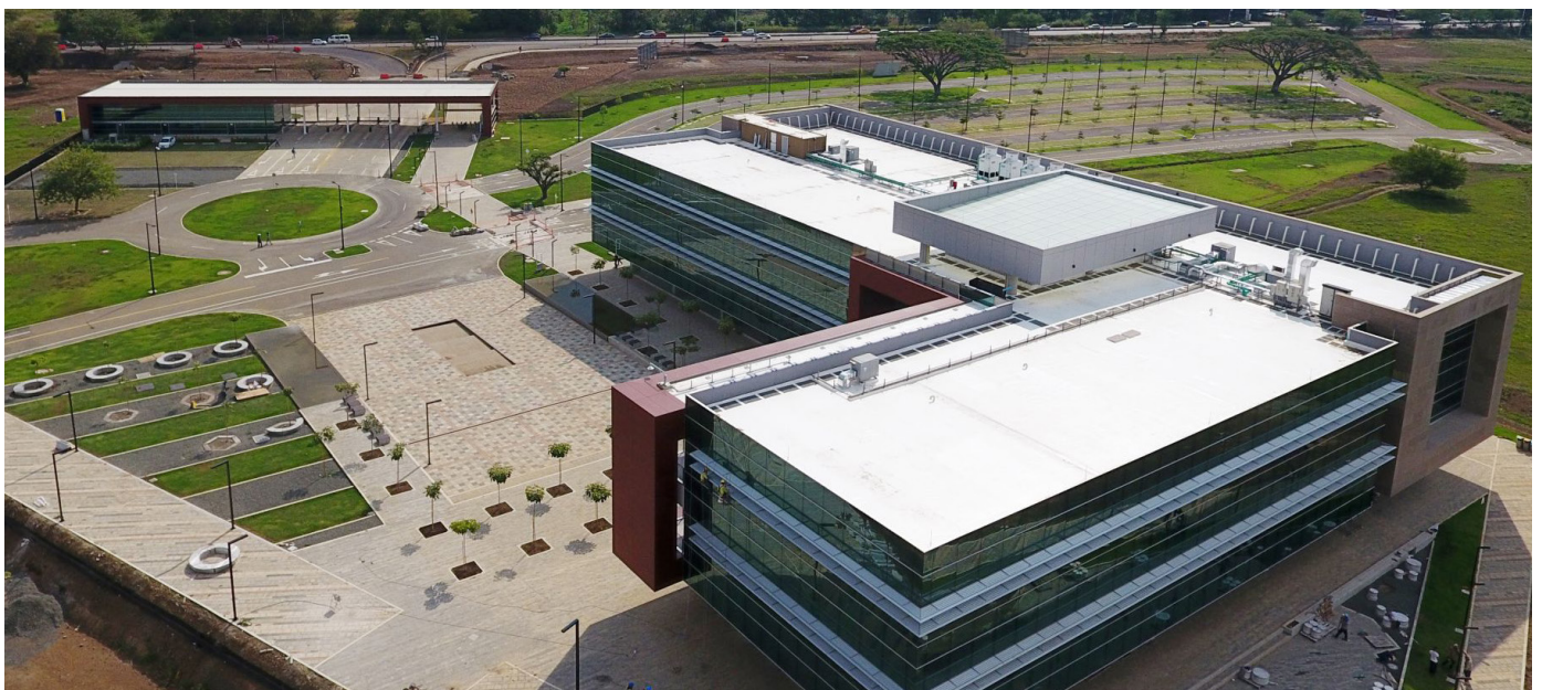
Figure 12.23 Example of a high albedo roof finishing to reduce urban heat island effect.
