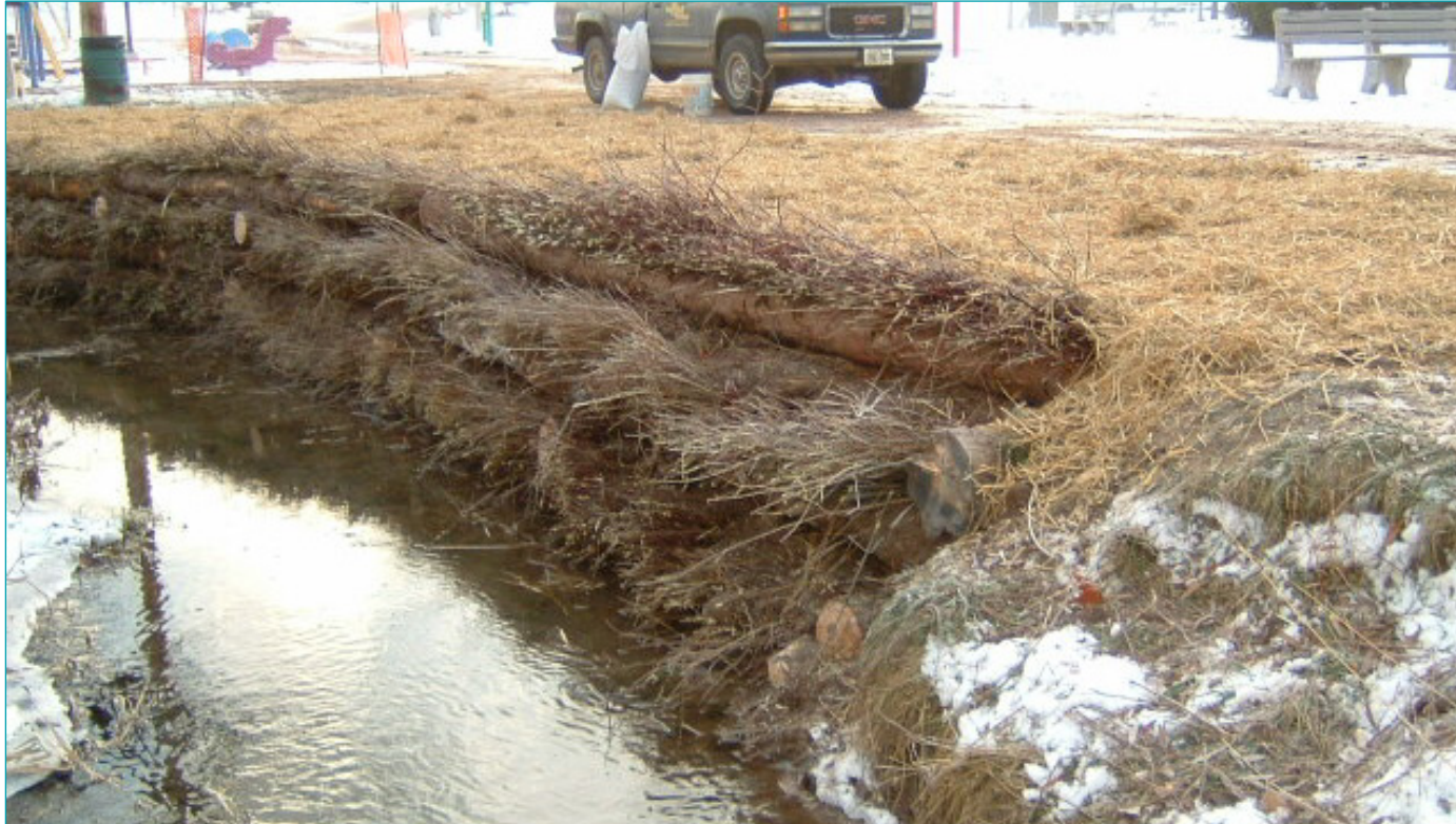
Timber crib bioengineered bank stabilization
