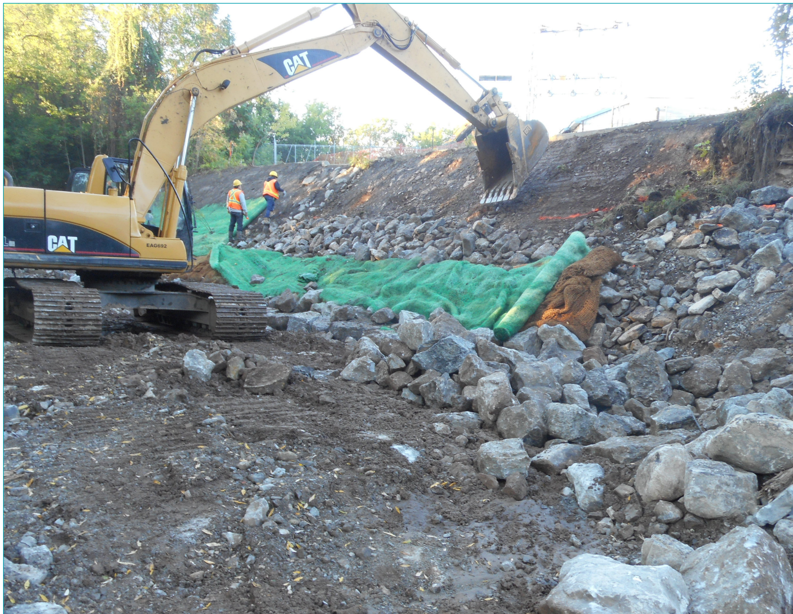
Typical creek bank stabilization with boulder revetment and vegetated banks
