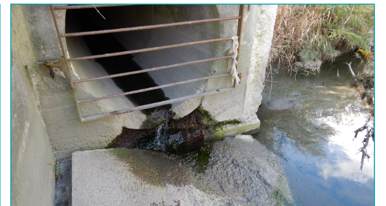
2 - The storm outfall and headwall structure has been exposed due to meander movement and widening. The northerly wingwall has failed and rests on the creek bed.
