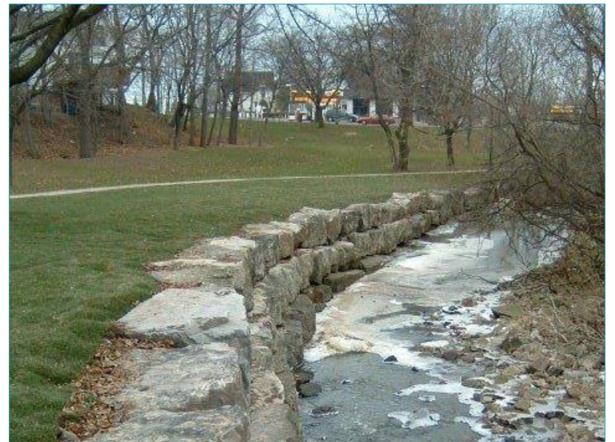
Rehabilitated creek bank with multiple rows of armour stone
