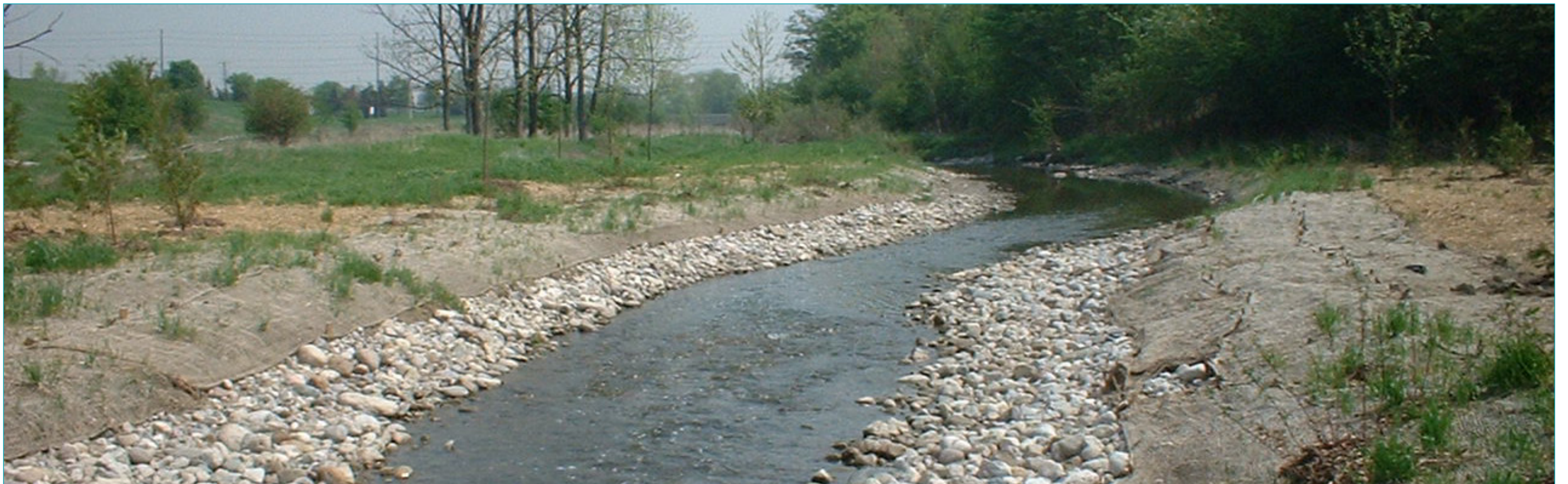
Full reconstruction and realignment of creek with natural stone pools and riffles, and vegetated banks
