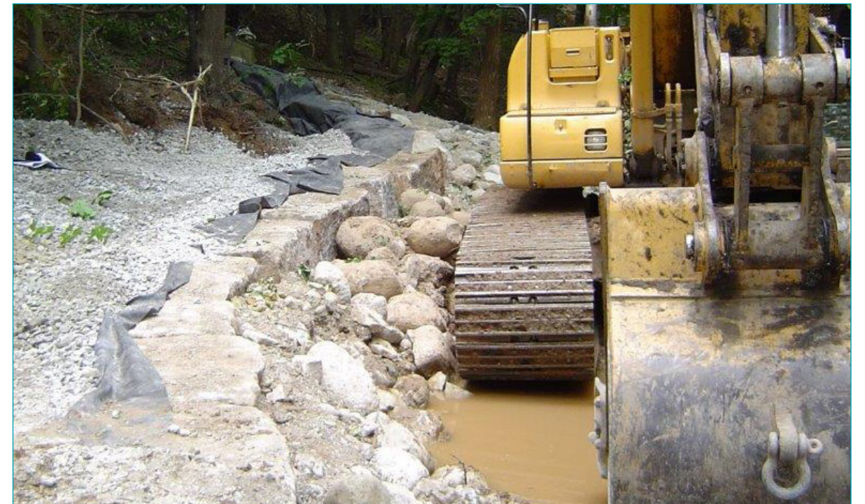
Boulder and armour stone bank stabilization
