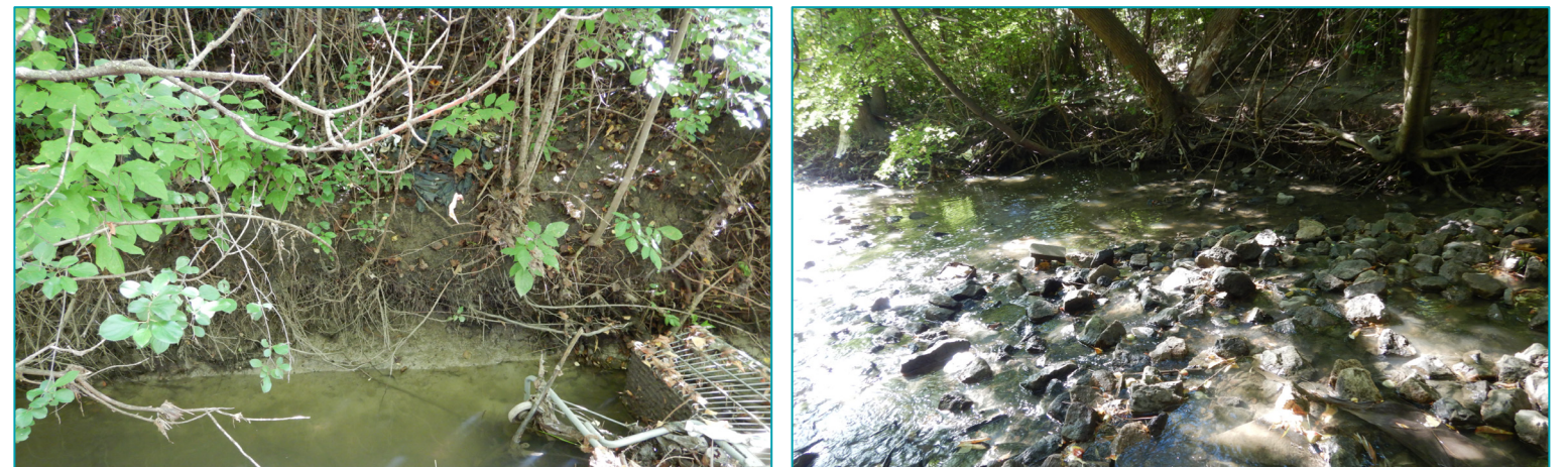
2 - Channel bank erosion has resulted in additional slope failure up the slope face and loss of vegetation.
