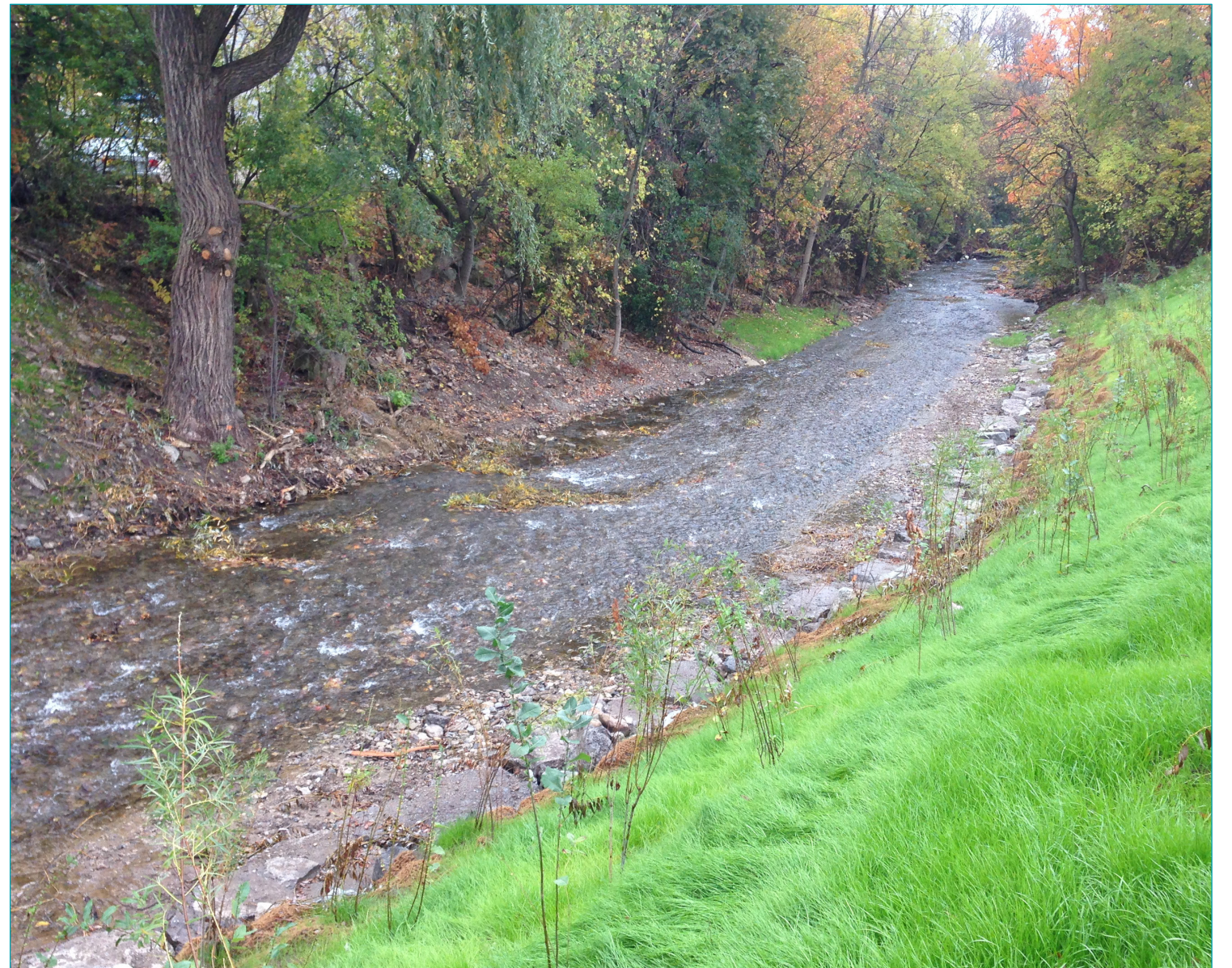
Rehabilitated creek with natural stone substrate, boulder toe protection and vegetated banks
