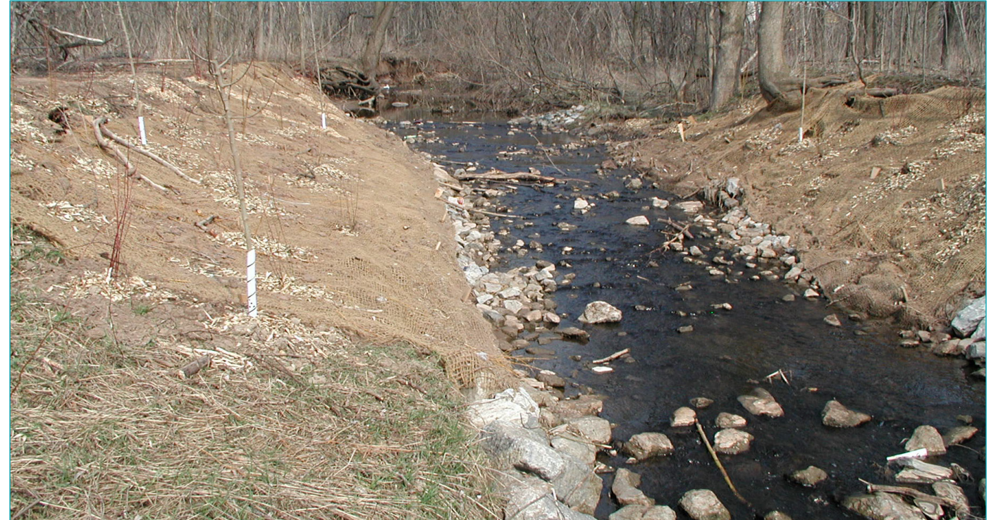
Localized erosion protection with minor regrading, stone and vegetated banks with erosion blanket
