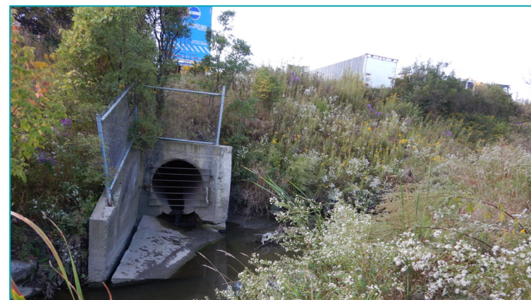
2 - The storm outfall and headwall structure has been exposed due to meander movement and widening. The northerly wingwall has failed and rests on the creek bed.
