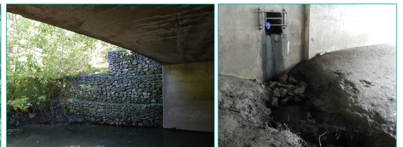
3 - Base row of gabions is failing along the low flow due to rusted wire. Erosion below the storm outfall.
