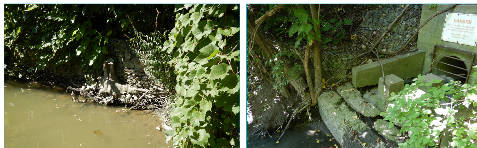
4 - The gabion wingwall is slightly undermined, and the base is sitting on soft saturated sediment.
