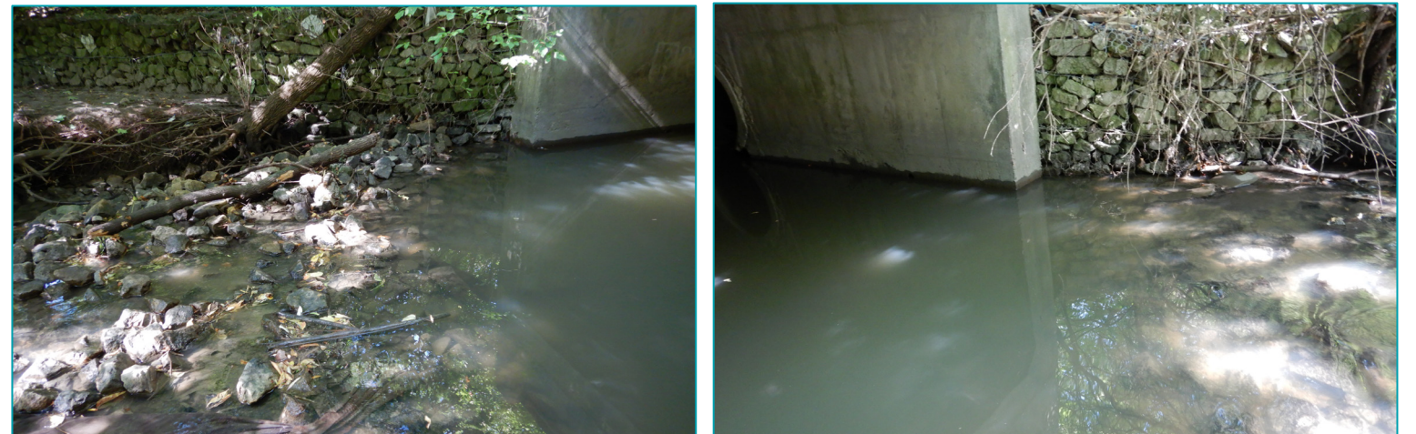
1 - The base or toe of each gabion has broken due to rusted wire and stone displacement has occurred.
