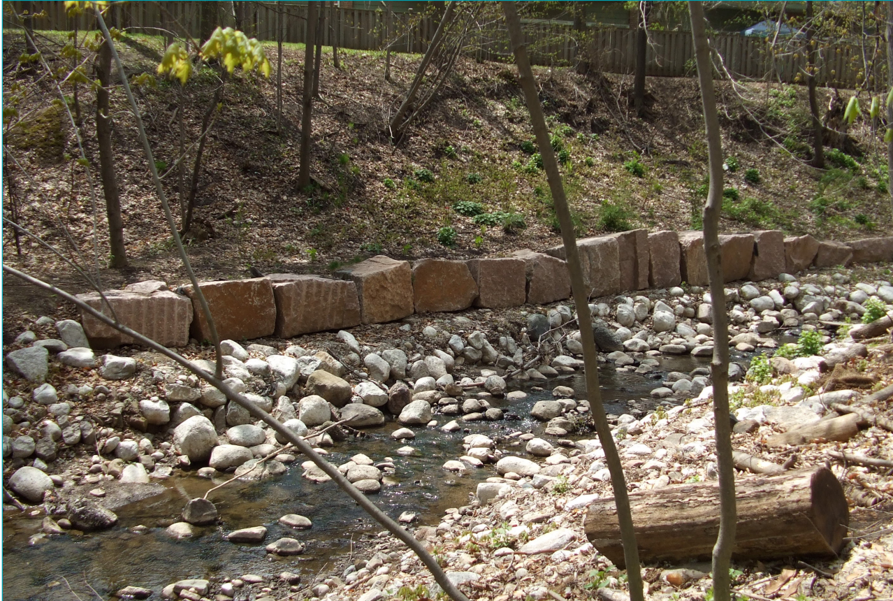
Creek with single row of armour stone
