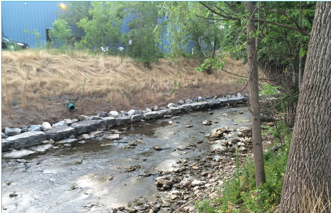
Boulder toe protection and vegetated banks
