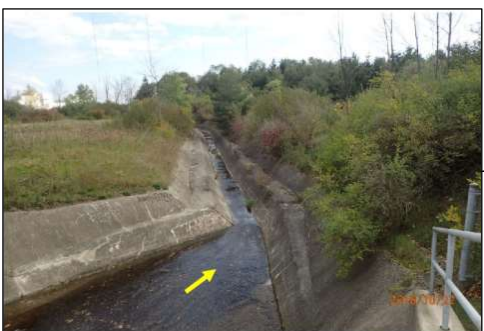
Clearview Creek downstream of Lakeshore Rd: concrete engineered channel
