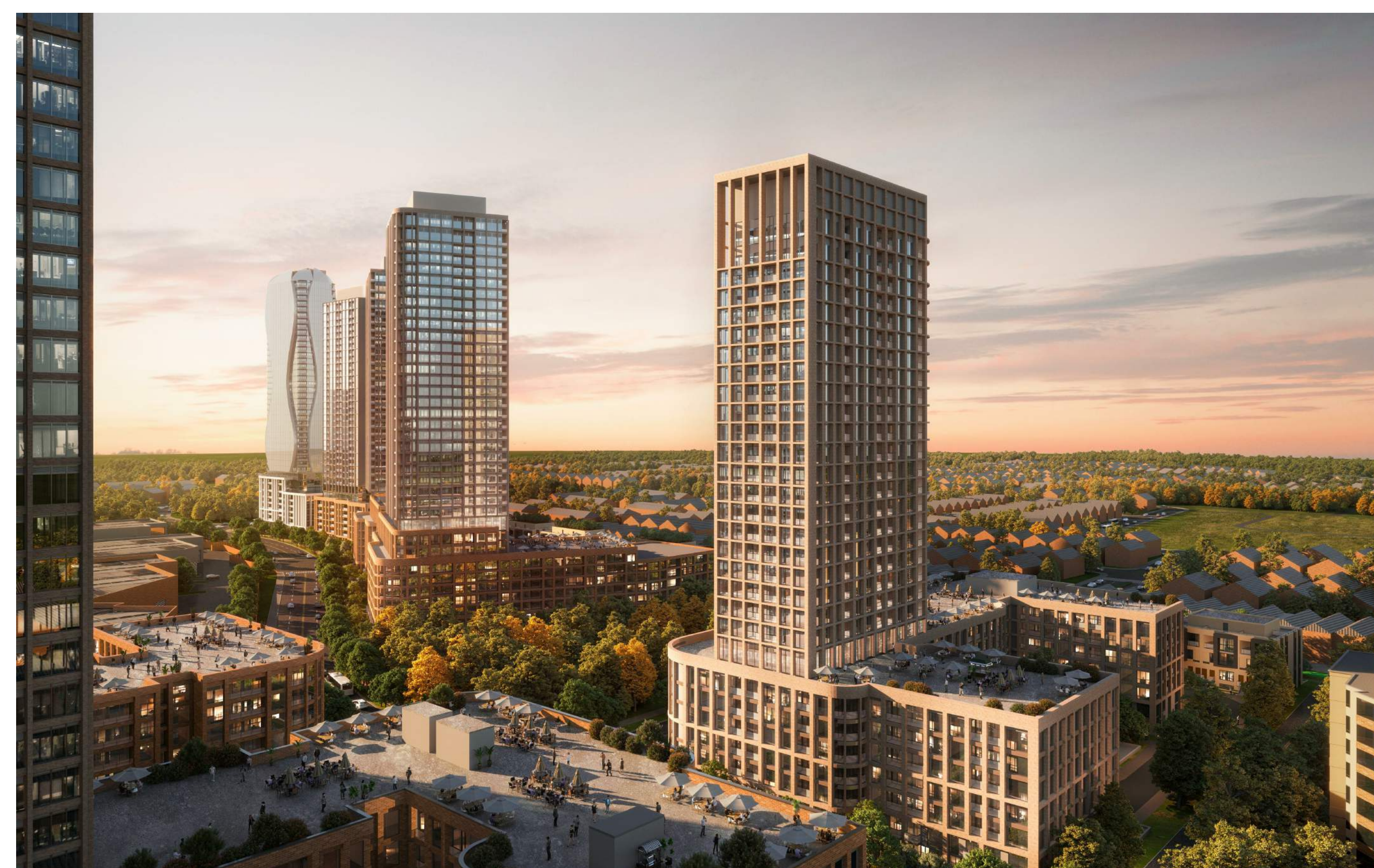
2 View from Acorn place North to Sorrento Drive A700.S
