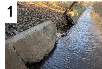
Broken concrete bank
