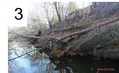
3 Failed gabion baskets
