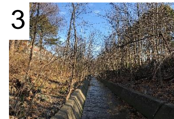
Flat wide concrete bed is a barrier to fish passage
