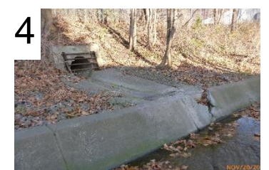
Cracked concrete bank
