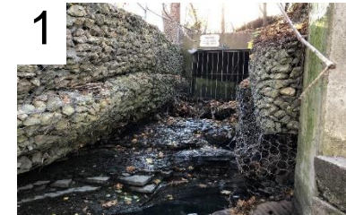
1 Scour of bed and damaged gabion baskets
