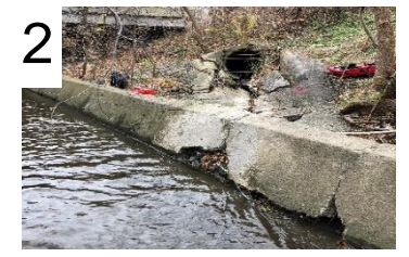
Broken concrete bank and outlet channel
