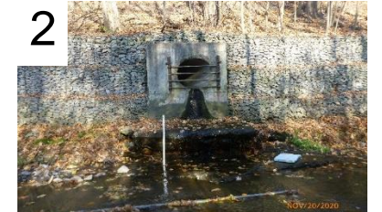
2 Downcutting of the channel bed
