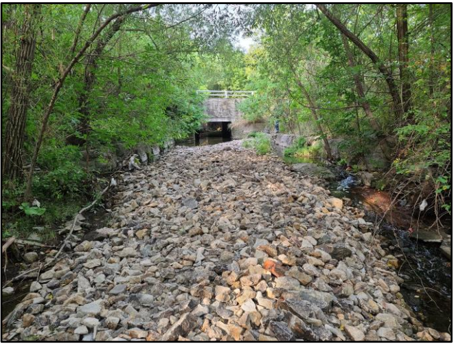
G. Large accumulation of engineered material, backwatering and impacting conveyance of culvert.
