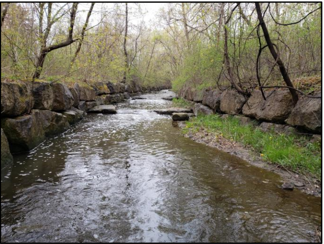
B. Section of armourstone retaining walls in fair conditions.
