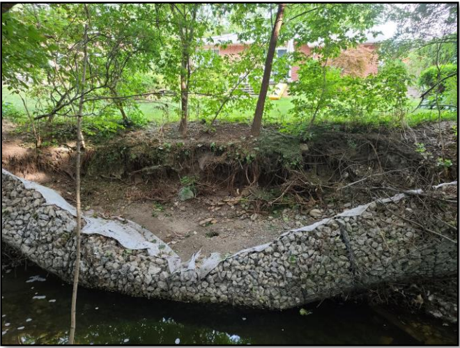
E. Failure of gabion baskets and loss of tableland in close proximity of private property.
