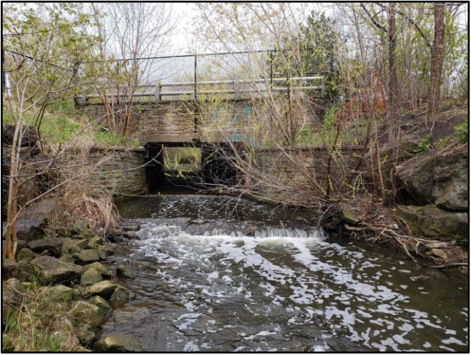
A. Upstream Thorn Lodge Drive culvert with brick-lined wingwalls in fair conditions.
