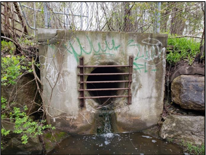
D. Existing deteriorated stormwater outfall immediately downstream of pedestrian bridge.
