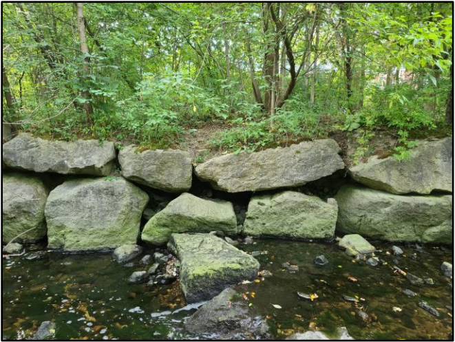
C. Section of armourstone retaining walls in poor conditions, with dislocated stone and loss of drainage material.
