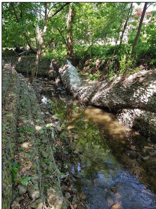
Photo 4. Failing gabion bank, north bank.
