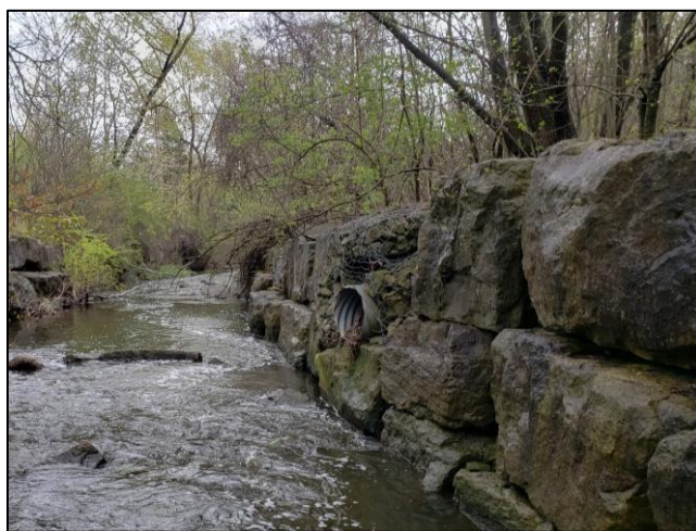
Figure 4-2. Deteriorated Stormwater Outlet Inset within Gabion Baskets Surrounded by Armourstone.
