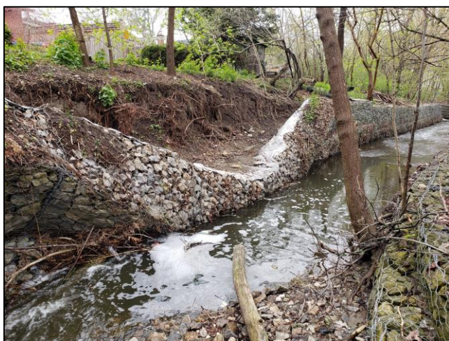
Figure 4-1. The Most Failed Section of Gabion Baskets within Study Area.
