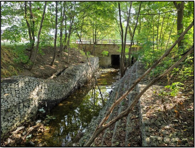
F. Failing gabion baskets with empty bottom, upstream of the downstream Thorn Lodge Drive culvert.
