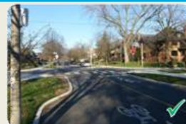
Reduced corner radii to slow down turning traffic
