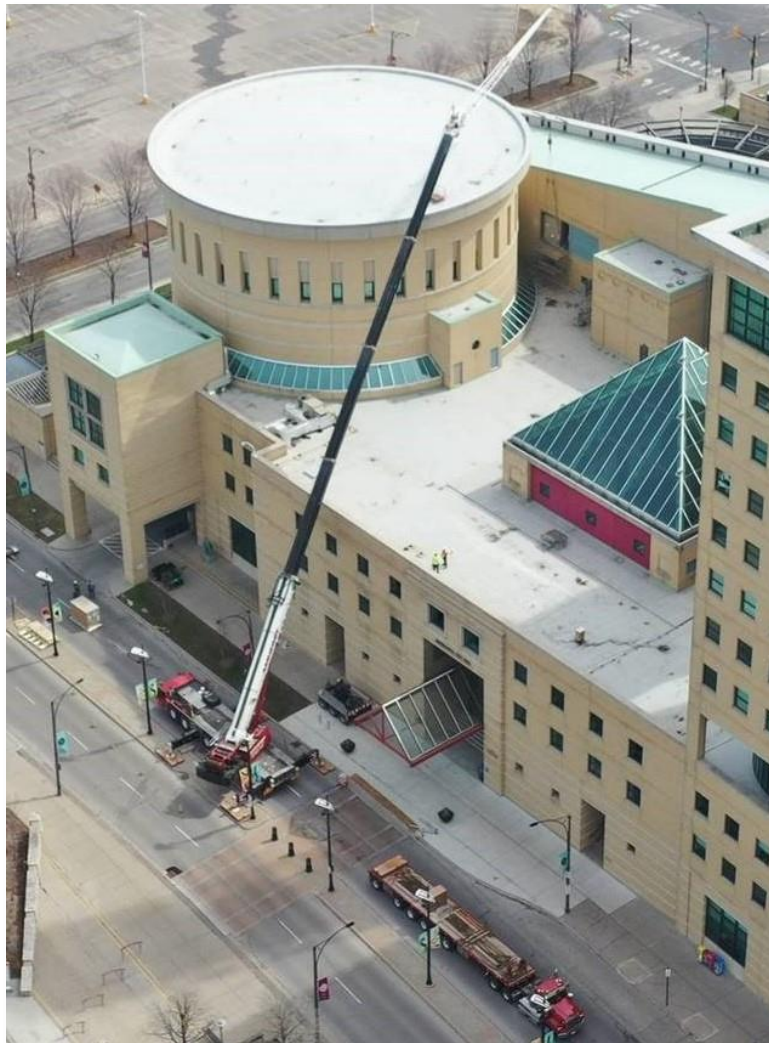
Mississauga City Hall AHU Crane Lift
