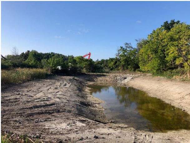
Sediment removal from stormwater management ponds near Old Derry Road in Meadowvale
