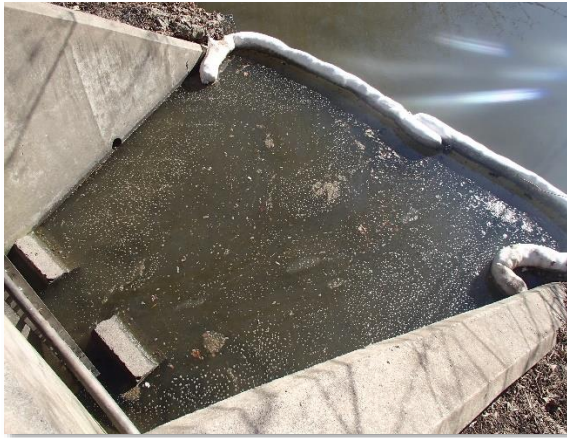
Spill containment from a storm sewer outfall to Lake Wabukayne
