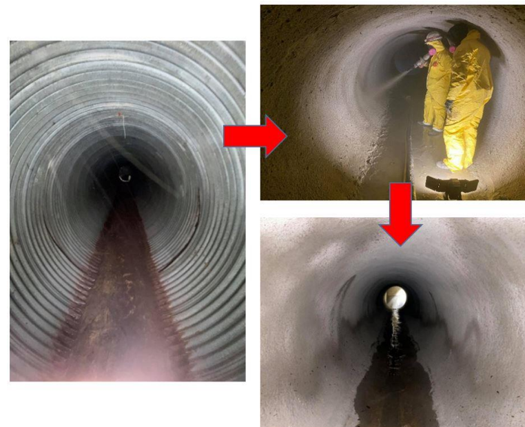
Rehabilitation of metal storm sewers using pipe lining technology
