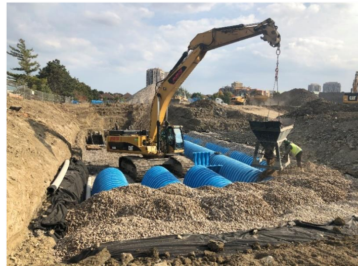
Construction of the Sandalwood Park underground flood storage facility in the Cooksville Creek watershed
