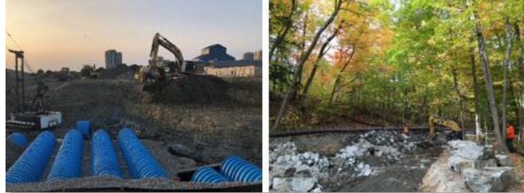
Construction of flood storage facilities and watercourse erosion control works are funded through the Stormwater Capital Program
