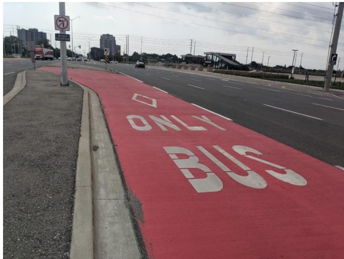
Red Plastic application on southbound Dixie Road to Transitway entrance
