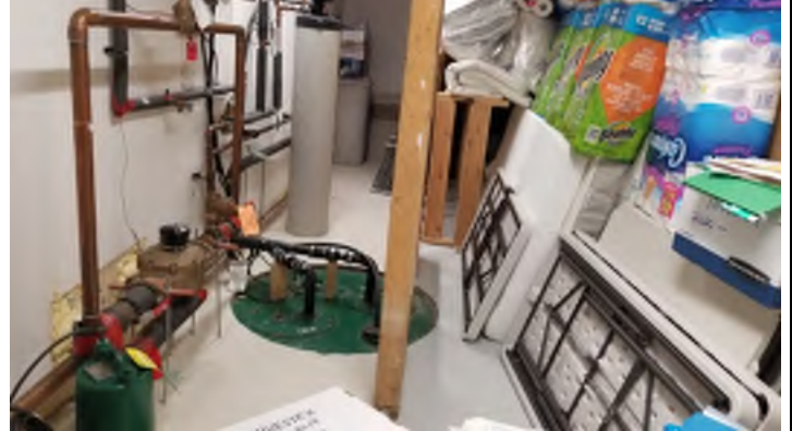
PHOTO 8: Sump pump in basement.
