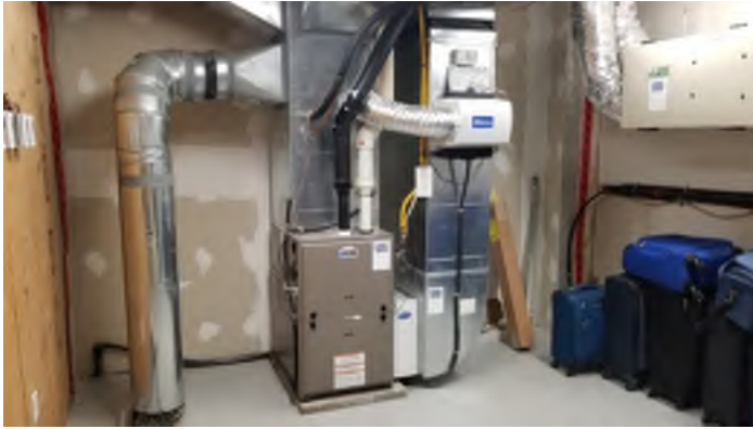
PHOTO 7: Natural gas-fired furnace in basement.
