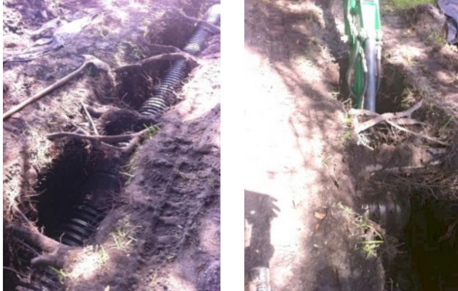
Fig 1. Utility installation below root system.
