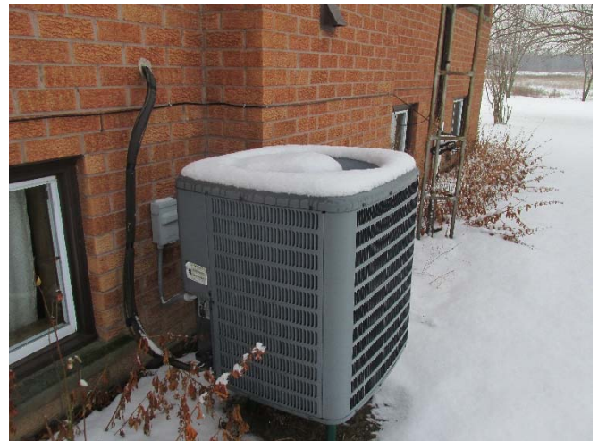
Photo 12: View of the ground-mounted exterior AC unit on the north side of the Subject Building.
