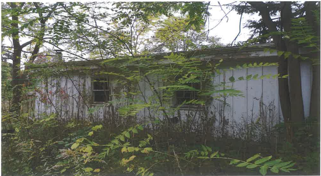
General view of Garage structure (looking northwest)
