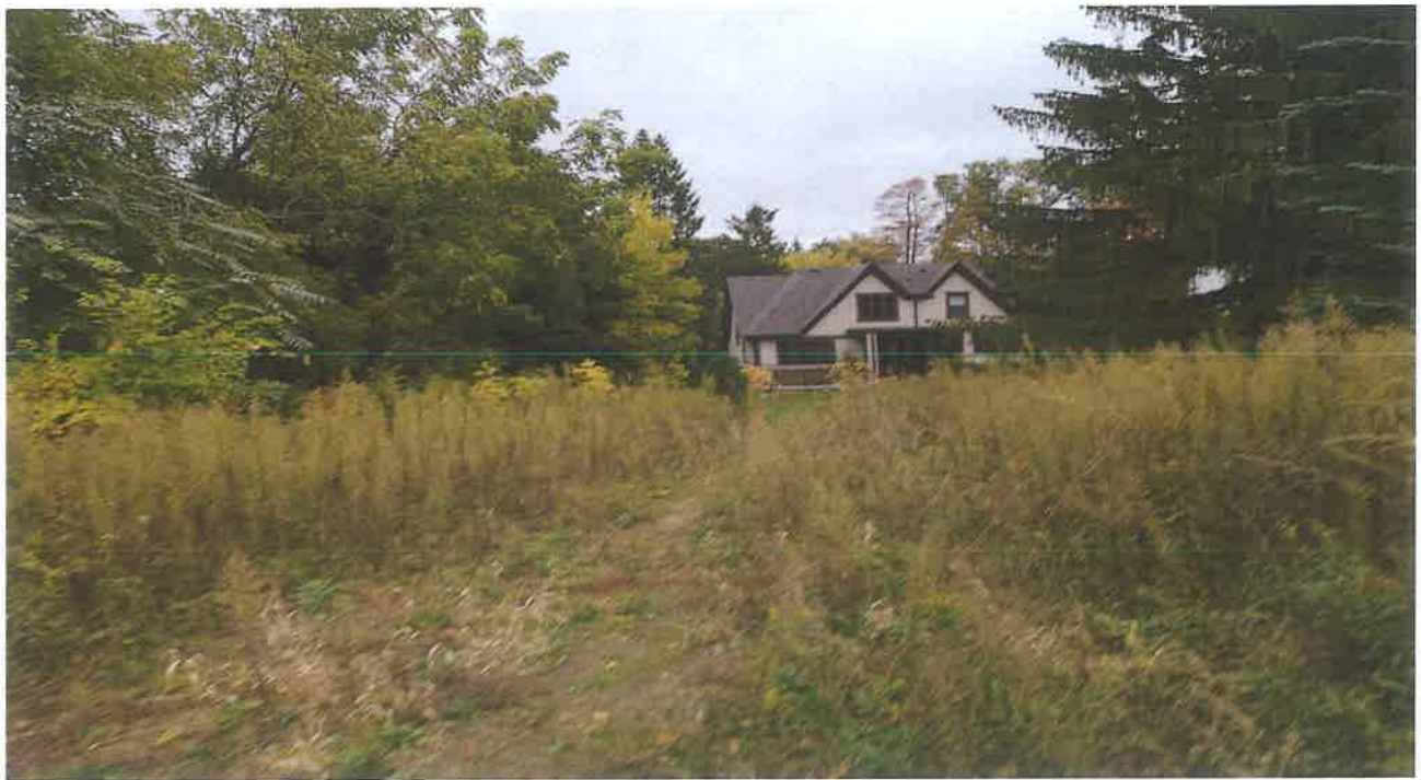
General view of subject site with neighboring structure (looking northeast)
