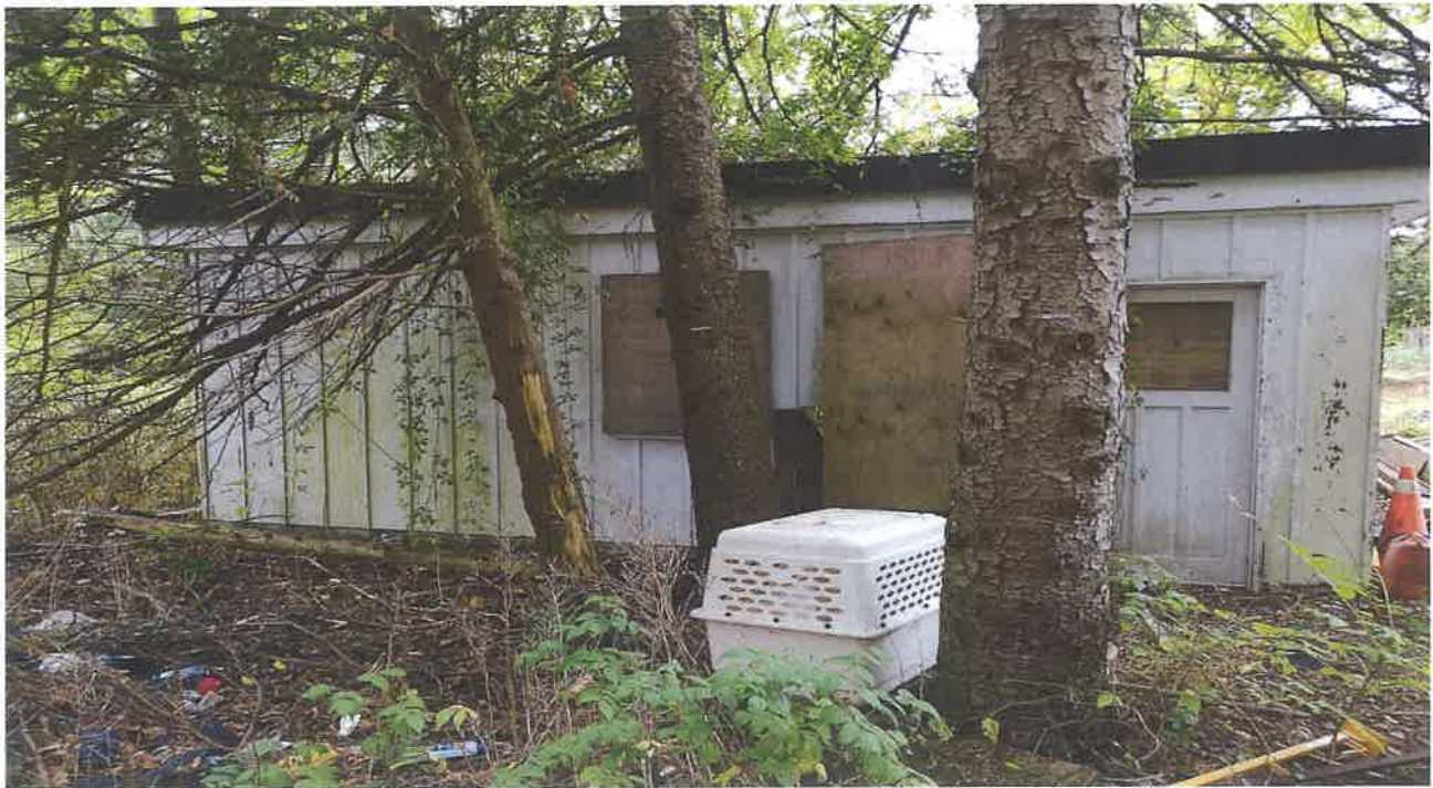
General view of Garage structure (looking south)
