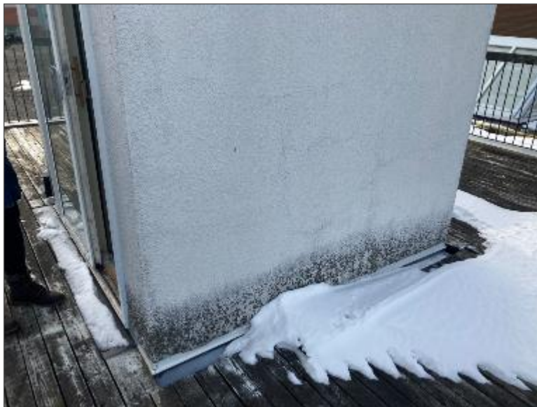
Photo 12 – Suspect mould observed on rooftop patio.
