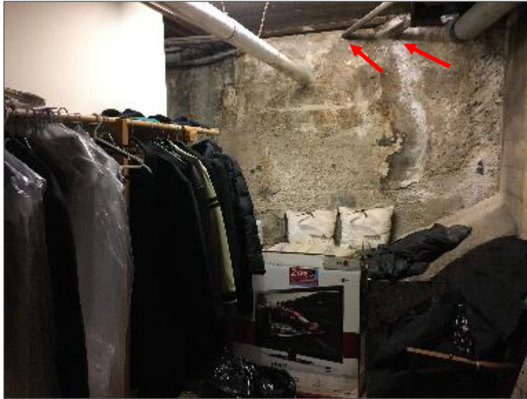
Photo 17 – Storage room, showing suspect vent and fill pipes.
