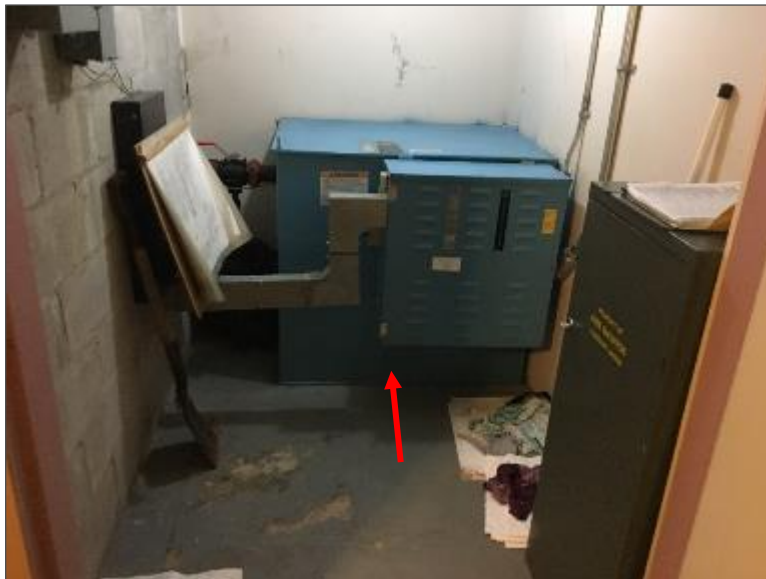
Photo 16 – Basement passenger elevator maintenance room, showing steel reservoir.
