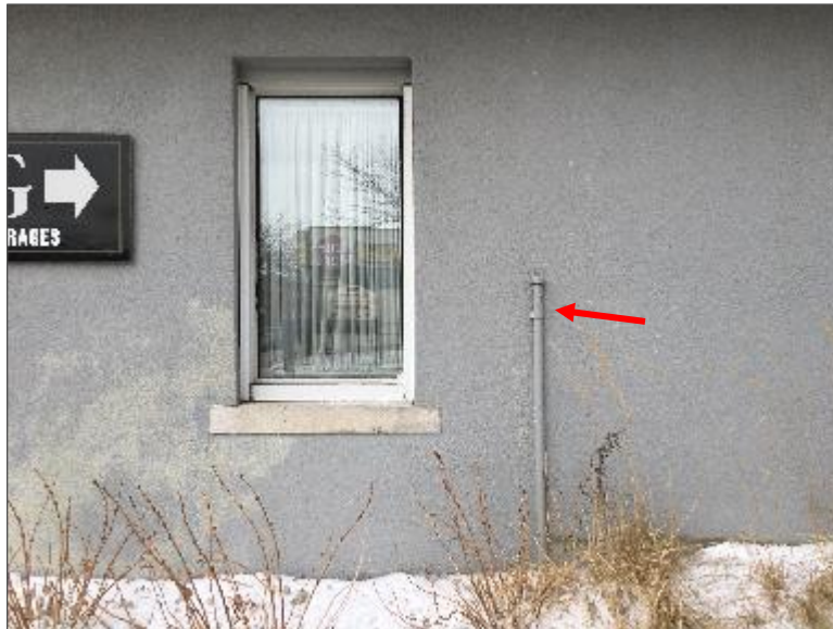
Photo 19 – Suspect vent pipe on Site Building northeast exterior wall.
