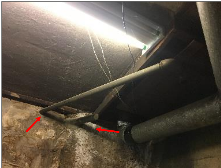
Photo 18 – Suspect vent and fill pipes in basement storage room.
