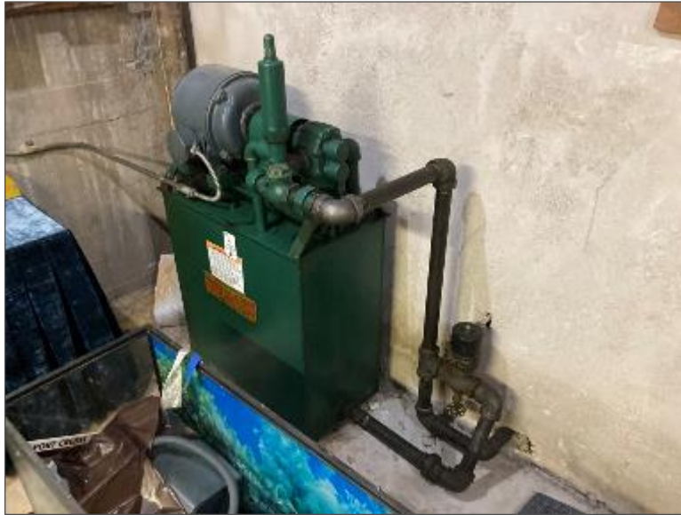
Photo 15 – Hydraulic reservoir for out-of-use freight elevator.
