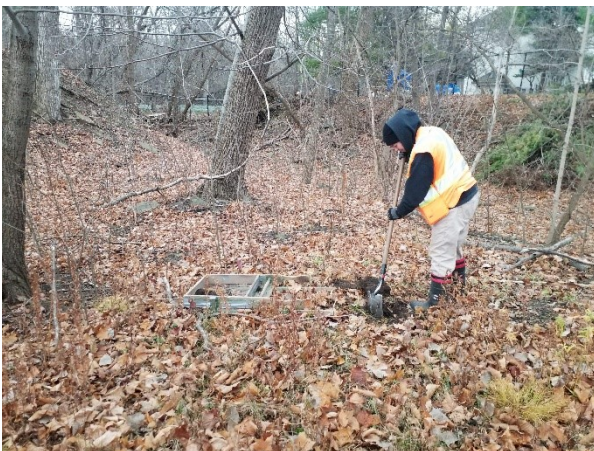
Plate 17: Crew test-pitting at five metre intervals.
