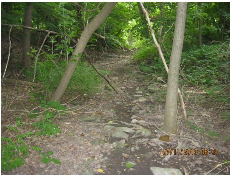
Photo 2. Looking upstream in the Old Sawmill Creek channel along the eastern extent of 2935 Mississauga Road, just upstream of the confluence with Credit River. Remnants of localized bed and bank armouring are present. Trees and shrubs have grown along the periphery of the engineered channel.
