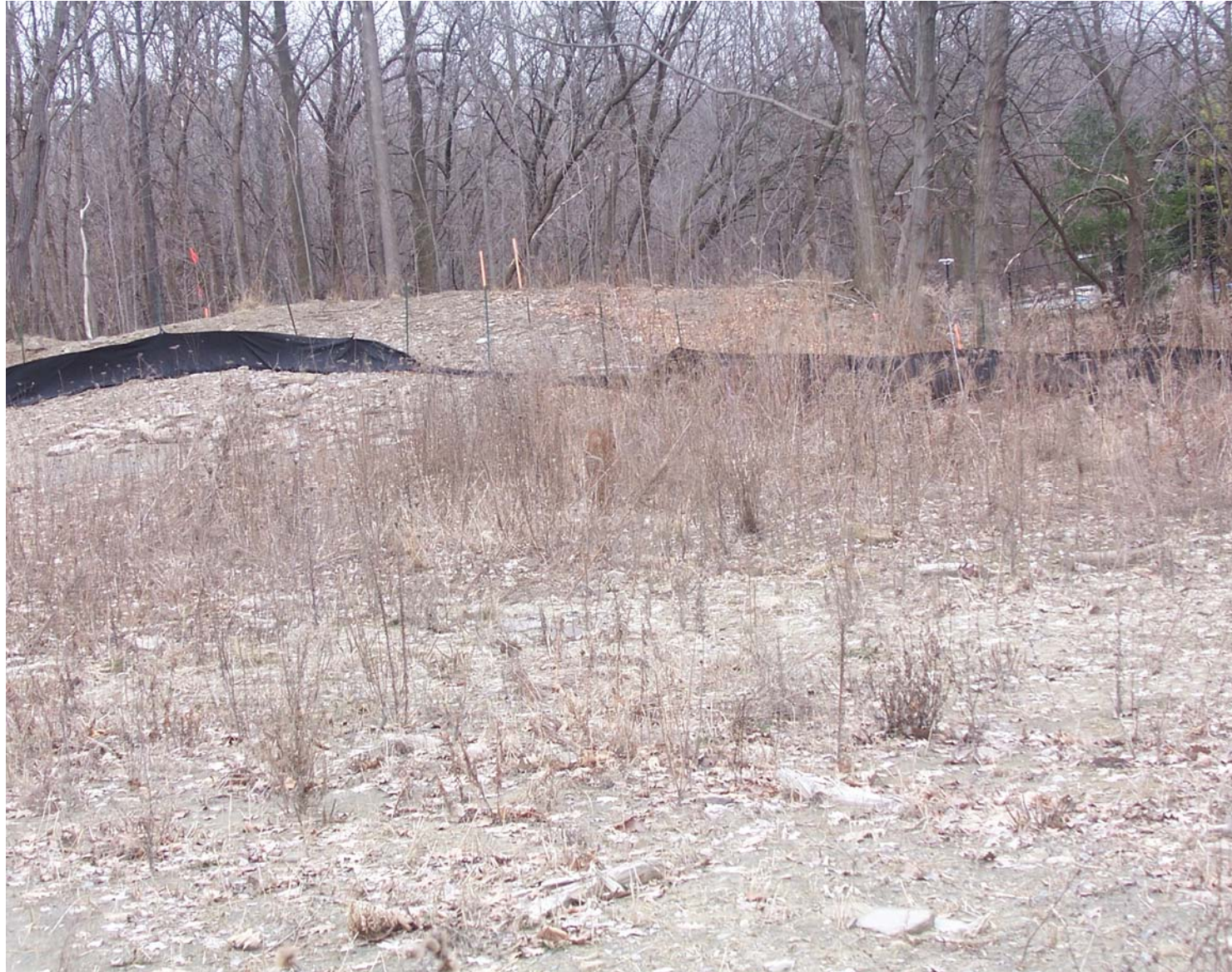
Photograph C: A view of southern portion of the site (inside the silt fence). This area includes patchy vegetation growth, and does not appear to include 'recent' fill.
