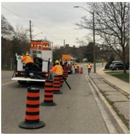
Installation of temporary active transportation lane
