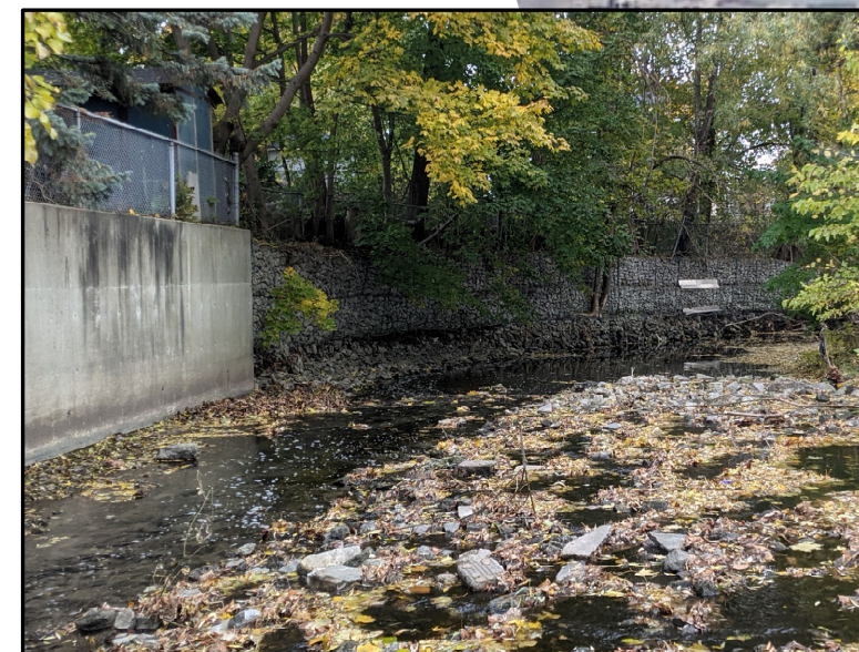
Downstream of Camilla Road Channel banks transition from concrete vertical wall to Gabion baskets (Looking Downstream facing East)
