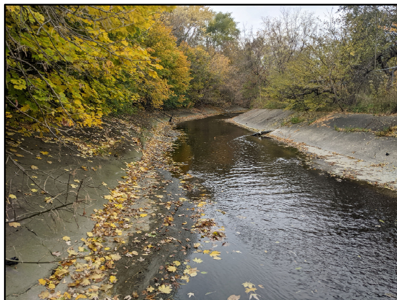
Upstream of Camilla Road Trapezoidal concrete channel (Looking Upstream facing West)
