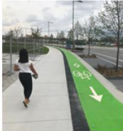
Continuous Detectable Tactile Buffer Strip, Vaughan
