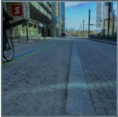
Detectable Curb Separation, Toronto
