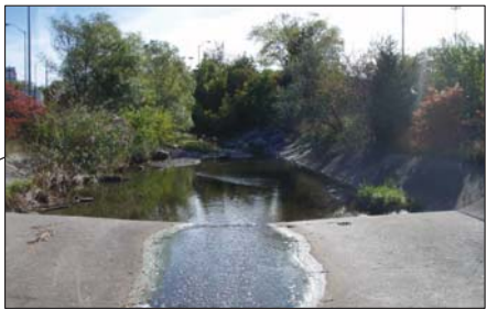
Sheridan Creek at CNR: concrete engineered channel
