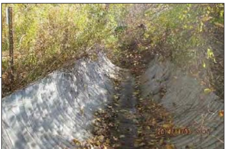
Avonhead Creek through concrete plant: CSP and concrete lined channel
