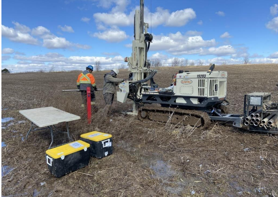
Photo 7: Geoprobe drilling borehole BH5-B beside groundwater monitoring well MW5-21.
