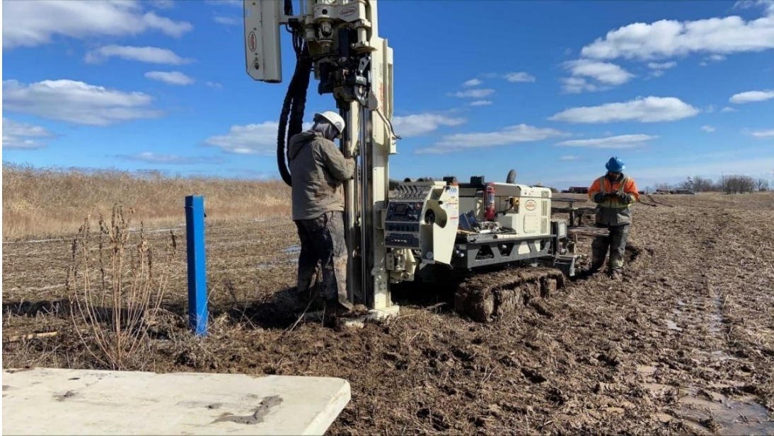
Photo 3: Looking southeast at Geoprobe drilling borehole BH1-B beside monitoring well MW1-21.
