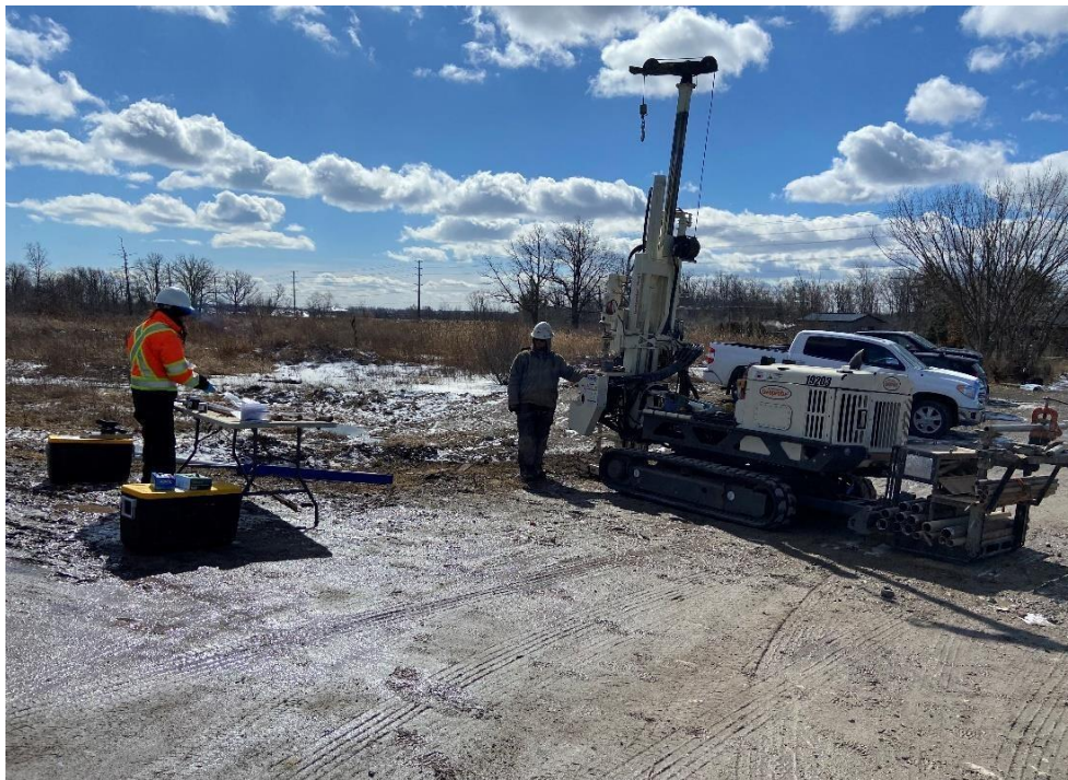
Photo 12: Looking south at Geoprobe drilling borehole BH-8 near east side of the Site.
