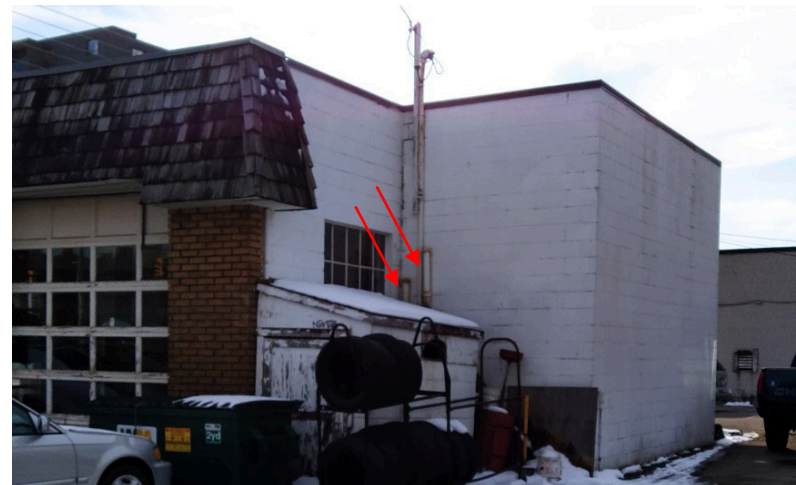
View of the vent and filler pipes (see arrows) associated with the aboveground storage tank at the adjacent property to the southeast.
