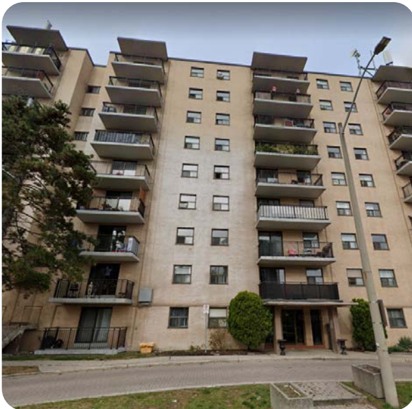
Figure 3: Existing Building at 3121 Kirwin Avenue, Google Maps 2021
