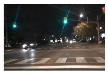
Figure 17: Traffic Signal Head with No Reflective Backboards
