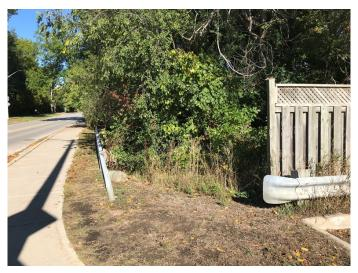
Figure 8: Guide Rail with Turned Down Approach End Treatment
