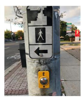
Figure 3: Non-AODA Compliant Pedestrian Push Button
