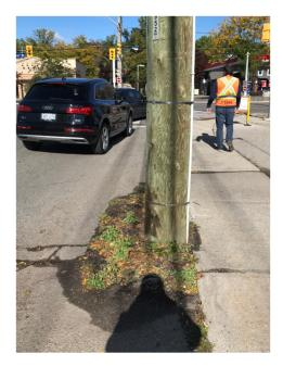
Figure 7: Pole located close to travel lane
