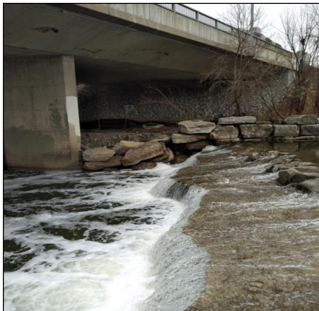
Figure 1.2 Scour Pool and Failed Armourstone Wall (April 2018)
