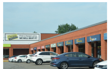
Figure 4.28 Retail Commercial buildings.
