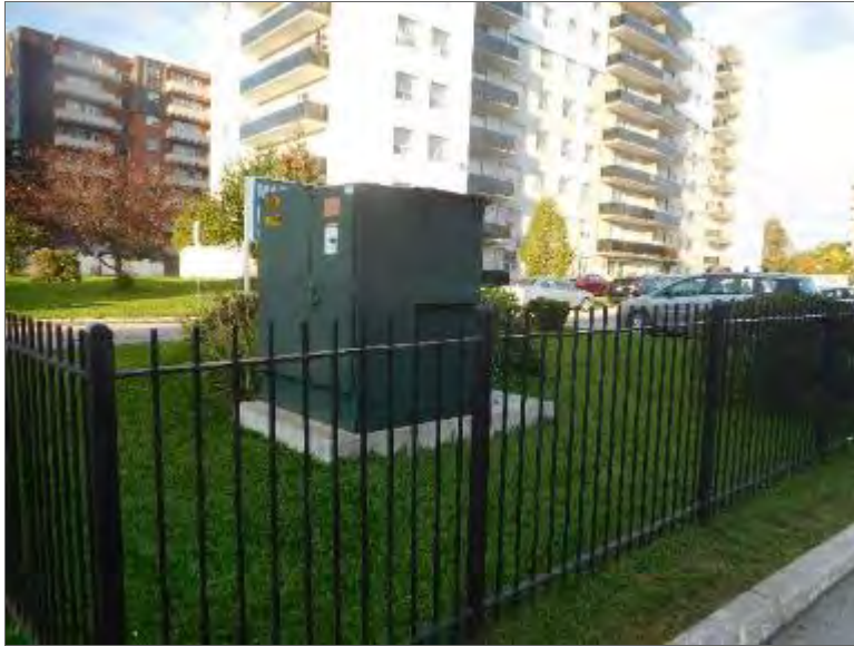
Photo 11 – Pad-mounted oil-cooled electrical transformer located in the southeastern corner of 1759 Bloor Street, looking west.
