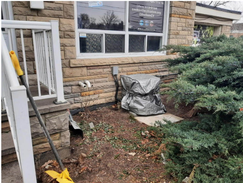
Photograph No. 6 – View of the furnace intake and exhaust pipes, and air conditioning unit located on the southwest elevation of the Site building.
