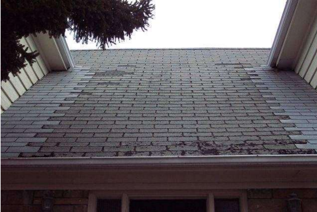
Shingle deterioration
