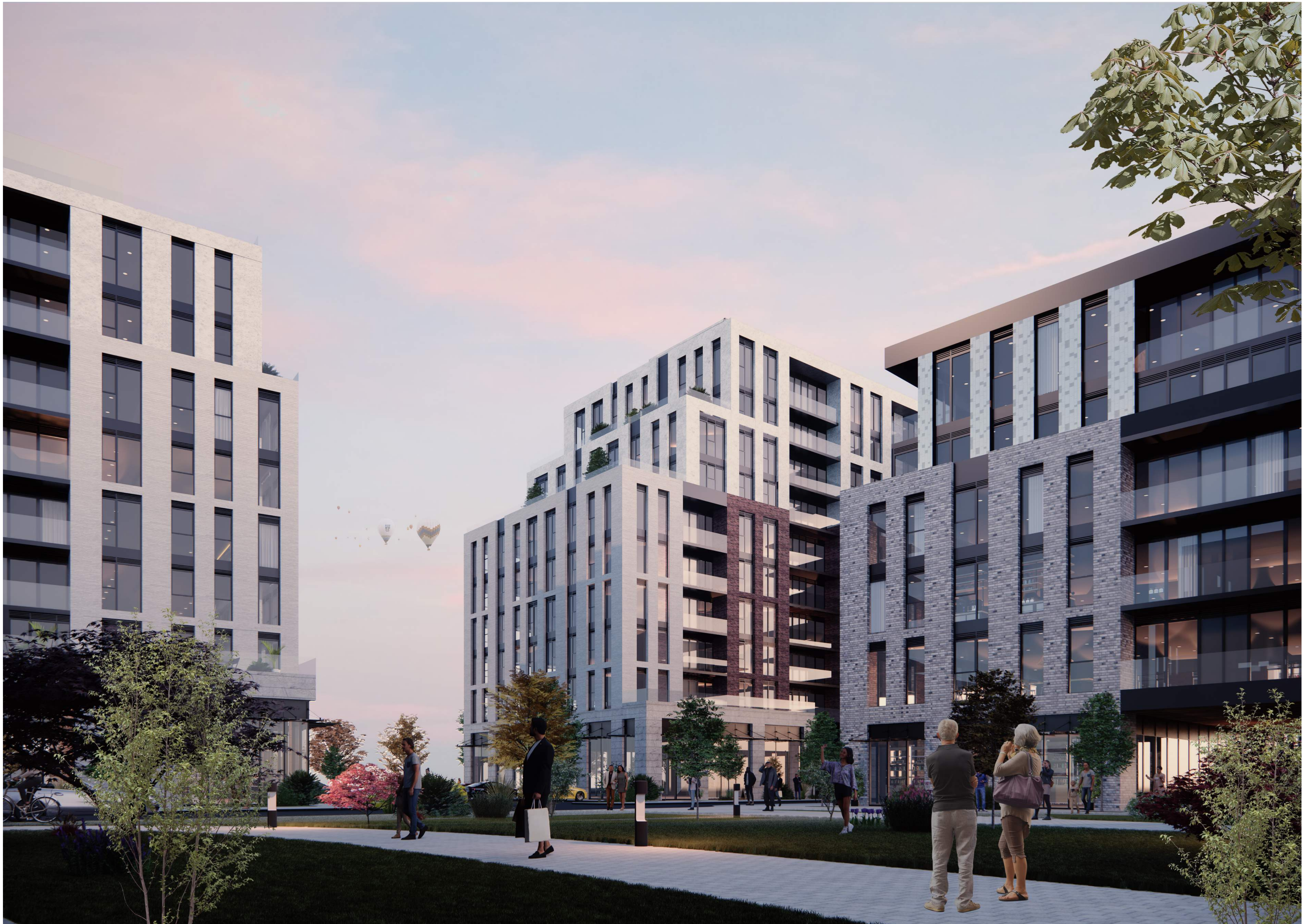
VIEW LOOKING AT BUILDINGS A,C&D FACING NORTH WEST
