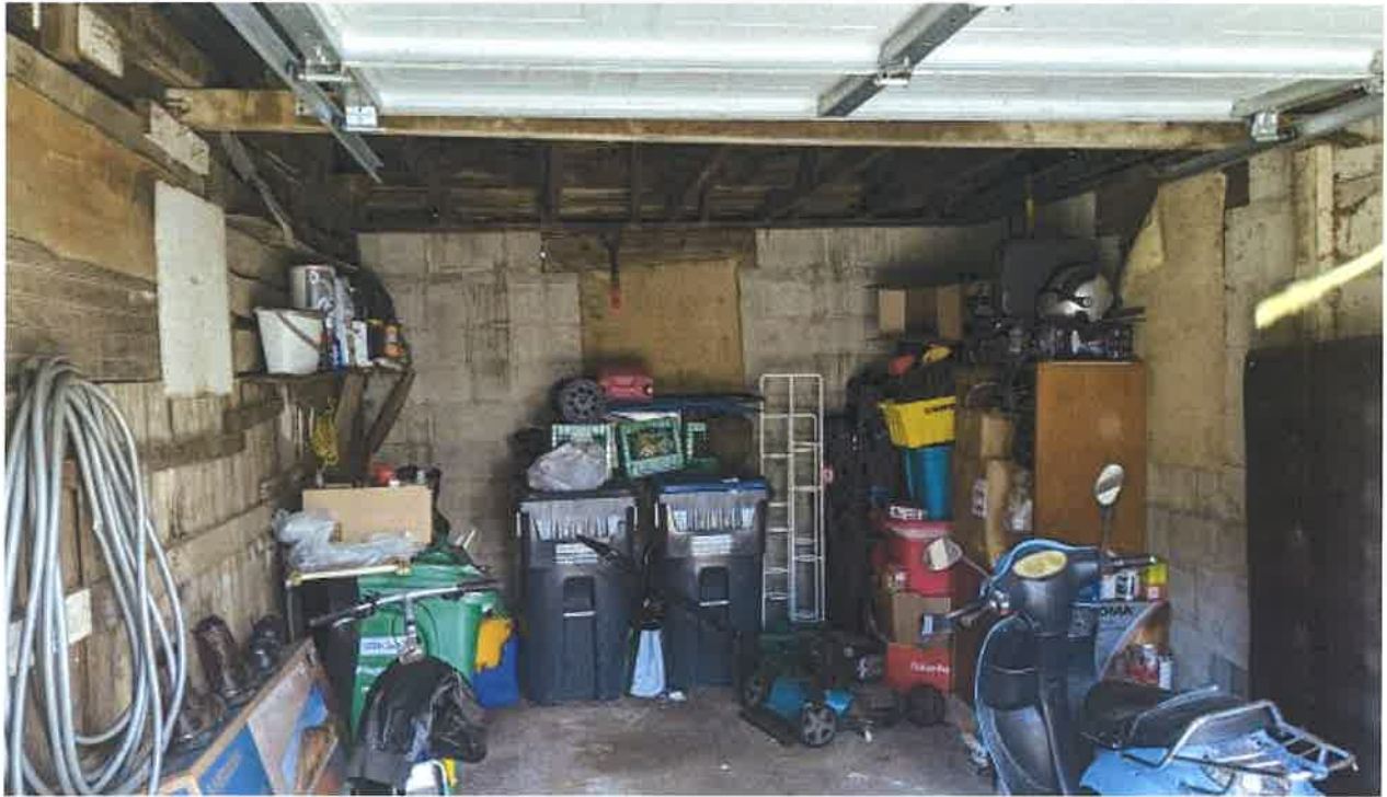
Interior view of the detached garage
