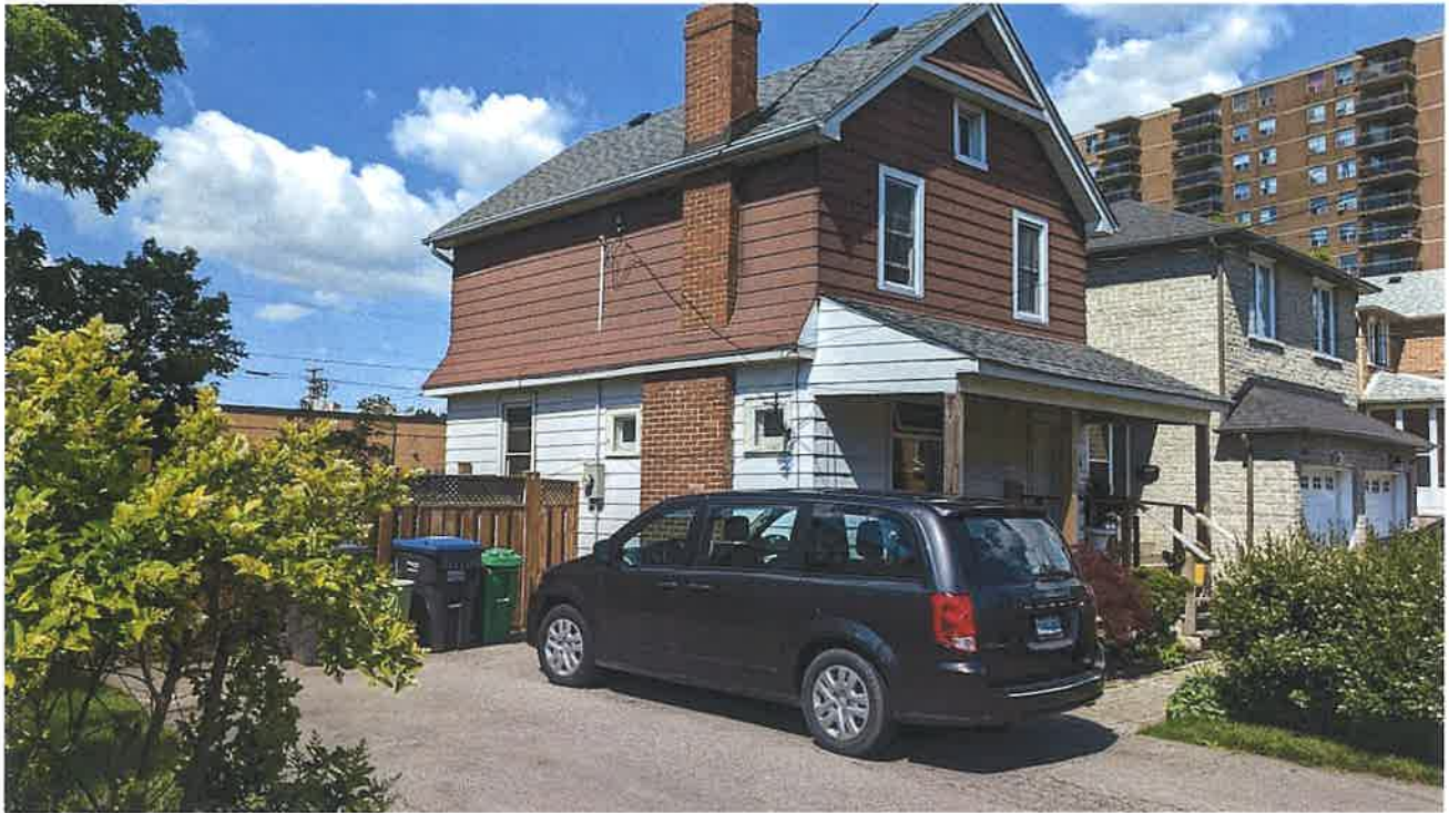
View of adjacent property to the northwest of the subject site (looking west)
