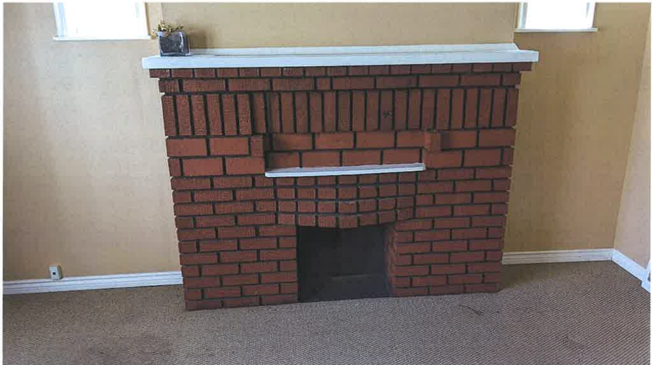
View of fire furnace located in the ground floor of residential building 1028 Caven Street
