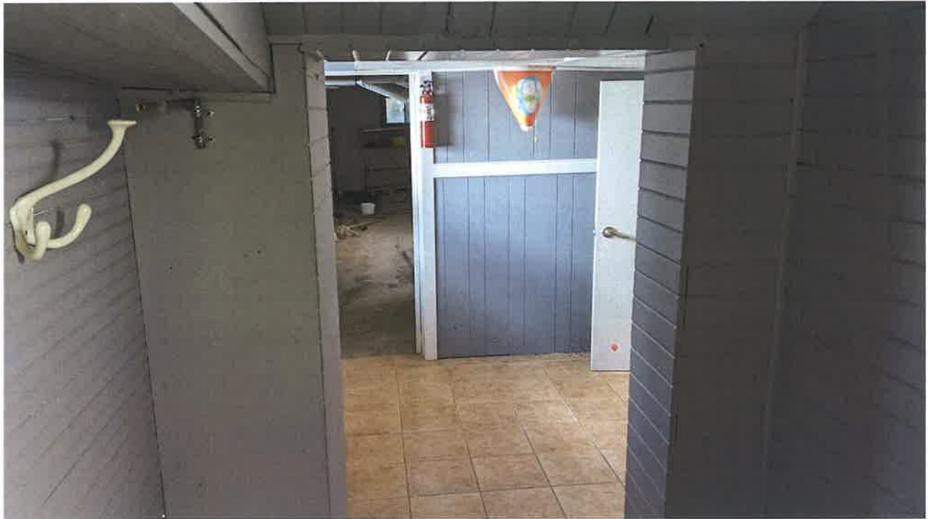
View of basement in the residential building at 1022 Caven Street
