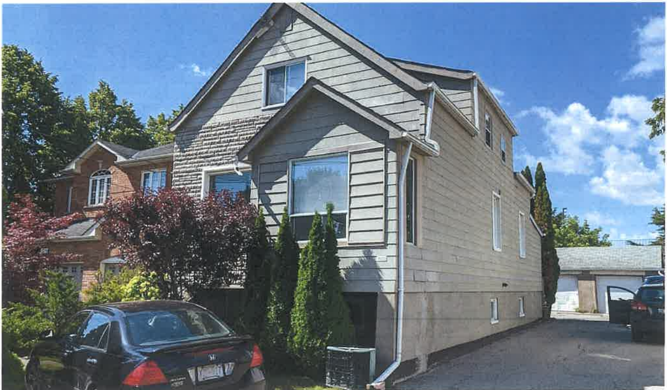
View of residential building at 1022 Caven Street (looking south)
